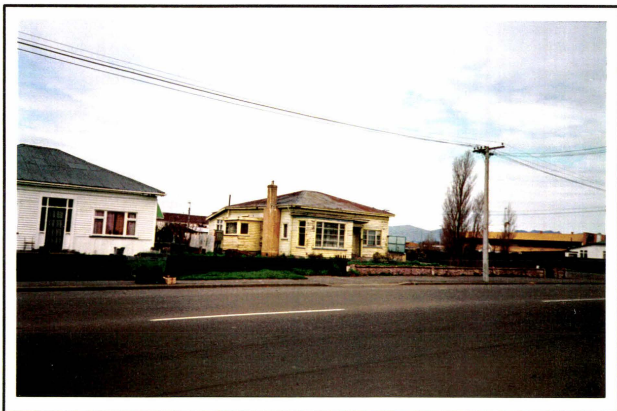
Planning Blight - Madras Street, St Albans, Christchurch - Many property owners along the proposed corridor of Christchurch's Northern Arterial motorway 'lost heart' in the maintenance of their homes. Nearly thirty years of uncertainty over the development of this project took its toll on the local environment and community.
