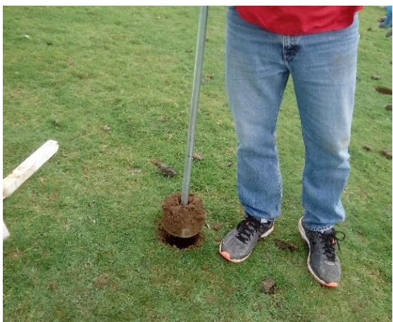
12. Drilling the hole
