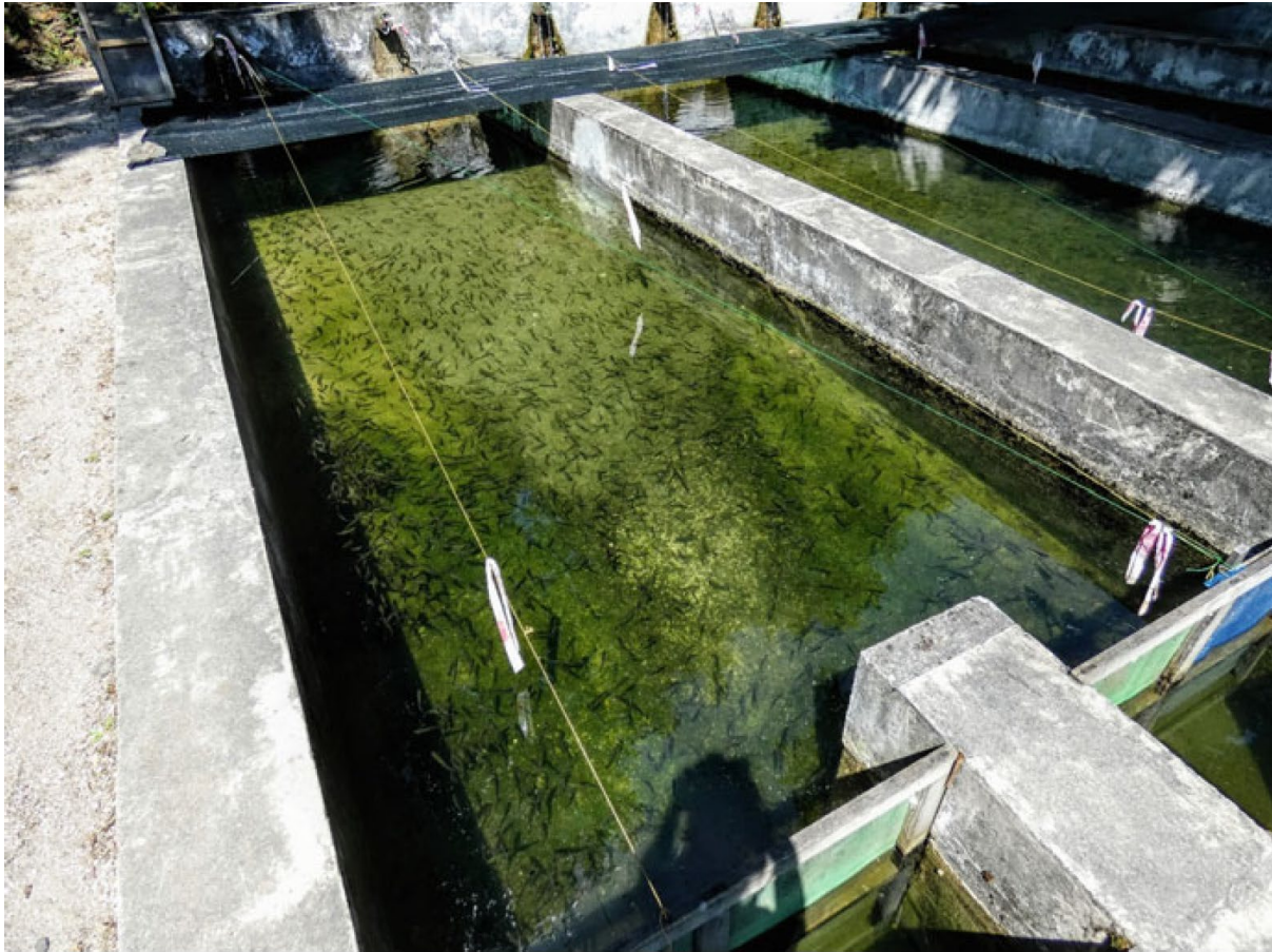
Figure 3. Concrete flow-through raceway in Norway. Similar style of flow-through raceways are used in New Zealand hatcheries. Reprinted by permission from Springer Nature Customer Service Centre GmbH: Springer Nature. Welfare of Farmed Fish in Different Production Systems and Operations by Hans van de Vis, Jelena Kolarevic, Lars H. Stein et al. Copyright (2020).
