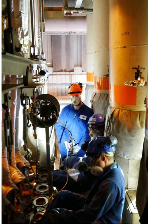
Figure 5: Inspection of a reformer tube during plant shutdown.
