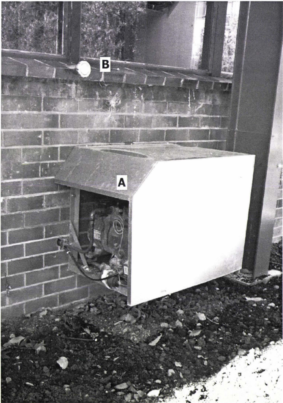
Figure 4.11: Photo of the refrigeration unit for the milk vat. [A] Refrigeration unit with shroud. [B] Exterior pipe to milk vat. Used to fill the milk vat from a truck parked outside.
