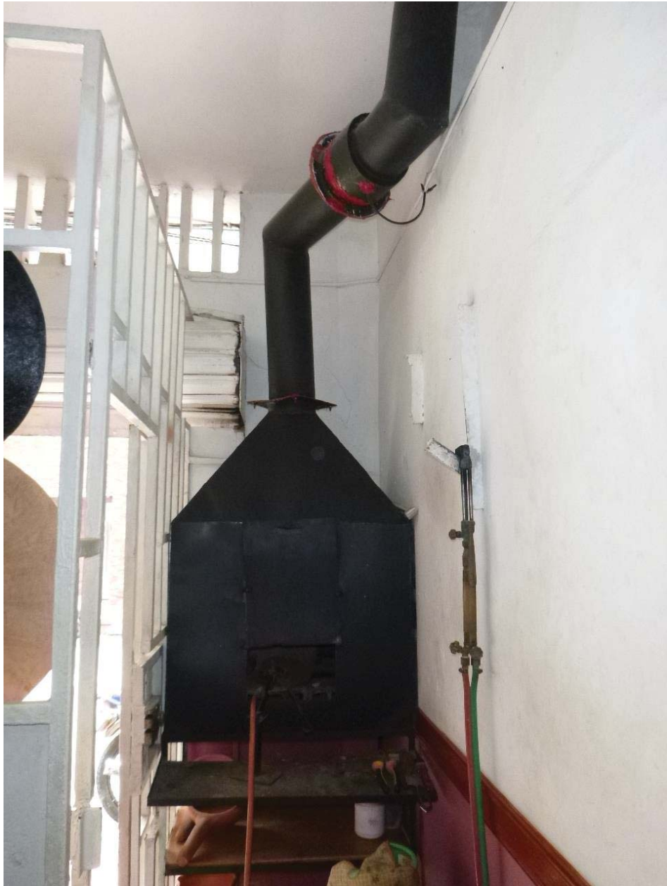
Figure 21: Fume hood leading to the retort.
