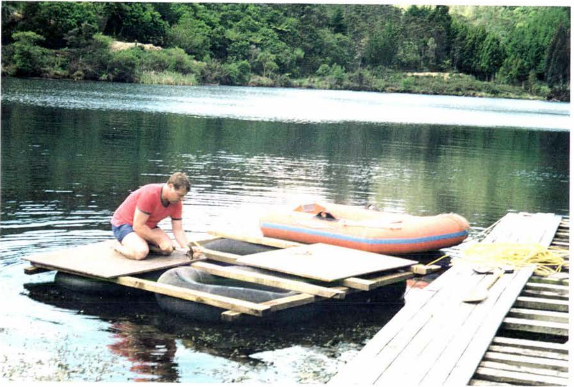
Figure 3.2 The raft used to core the deep water sites being assembled on the lake at Te Pohue
