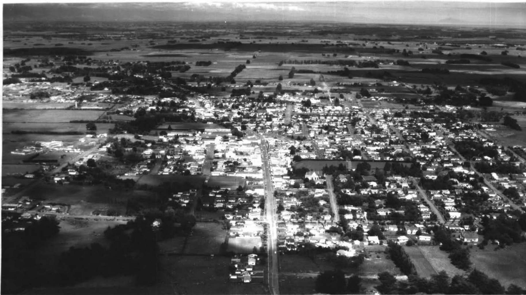
Plate 1: An aerial view of Marton, looking south. Part of Marton Junction is seen at the upper left of the photograph.
