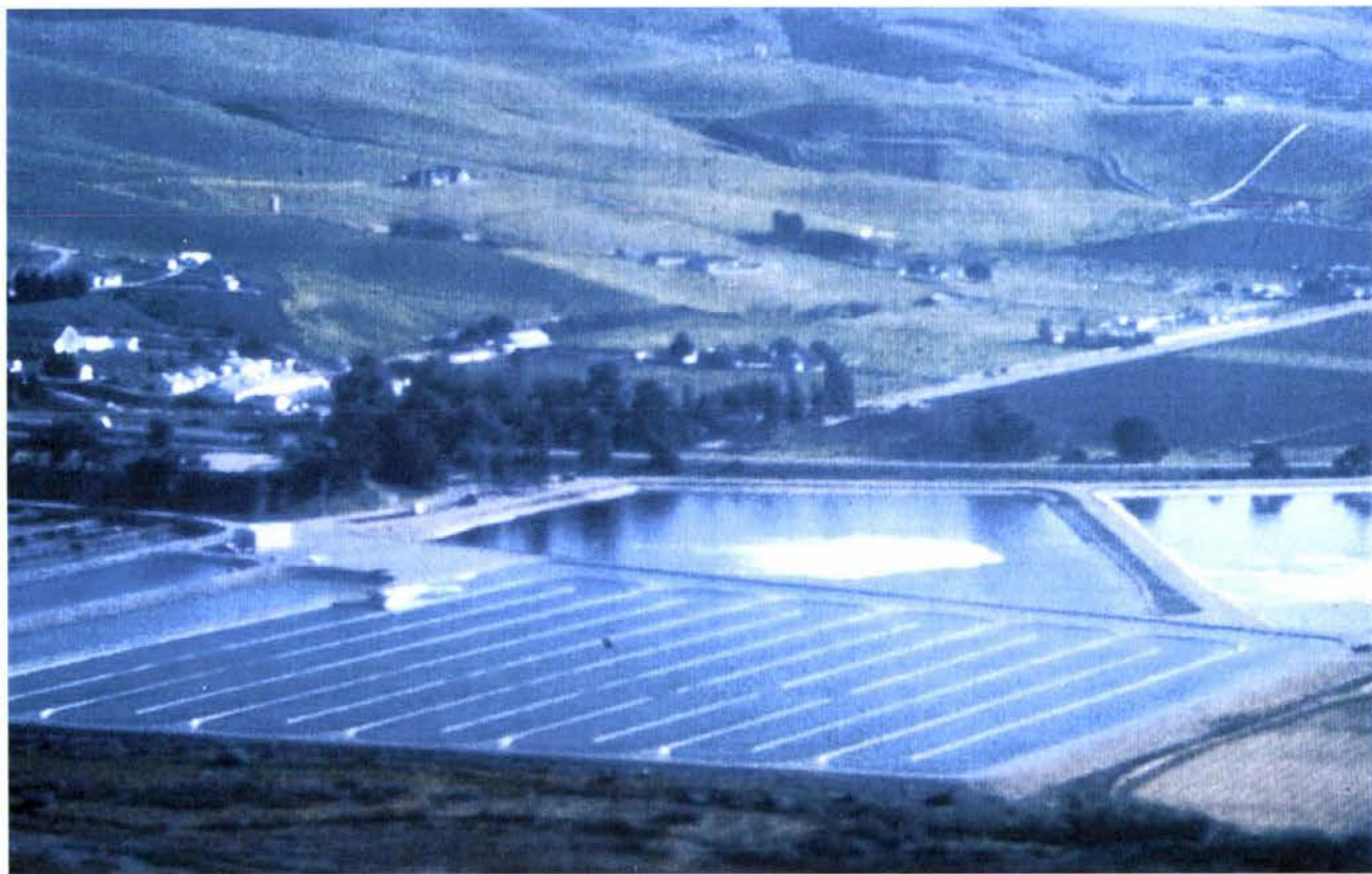
Figure 1.4: A large (~5 ha) paddle wheel mixed, meandering high rate algal pond treating municipal wastewater at Hollister, California (from Benemann 2003).
