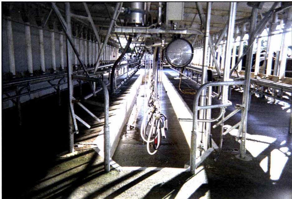
Figure 2.11: A simple high-line, swing-over Herringbone dairy
