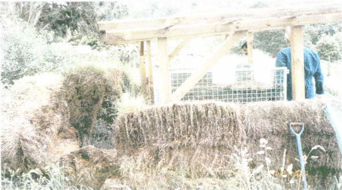
Fig. 4.7 East view of straw bale wall wind barriers.
