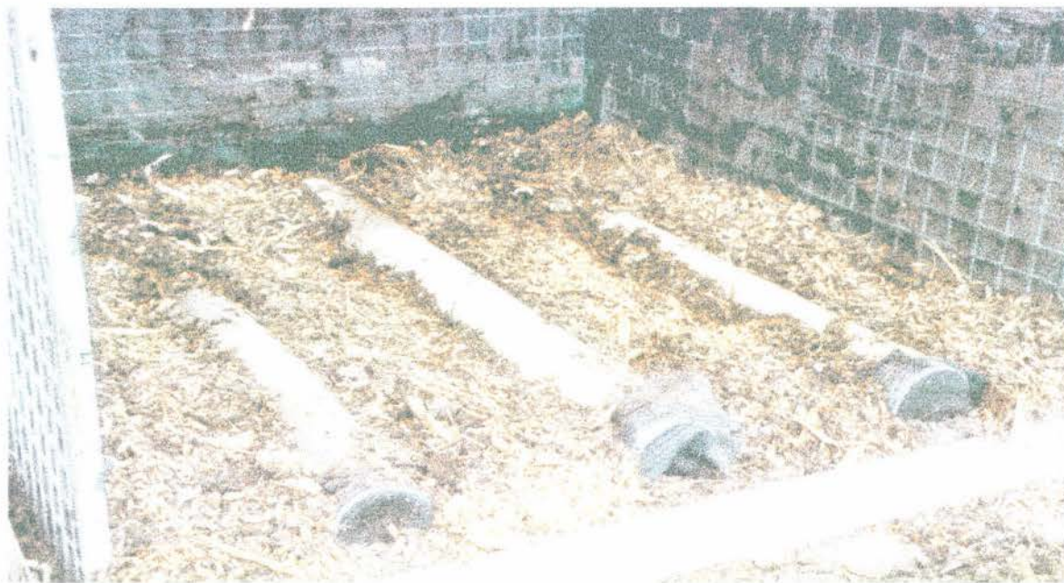
Fig. 4.2 The passive aeration pipes placed on a base material wood chips.
