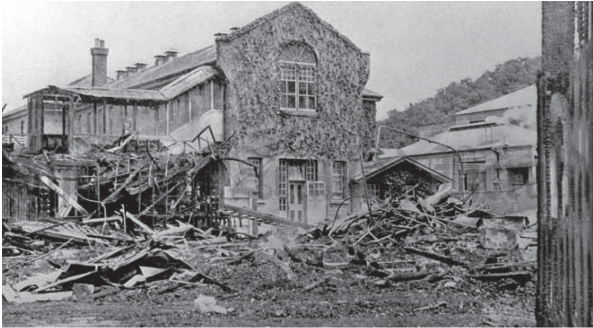
Figure 2 Seacliff Mental Hospital, Dunedin, pictured after the fire in 1942. Picture courtesy of Te Ara, Wellington
