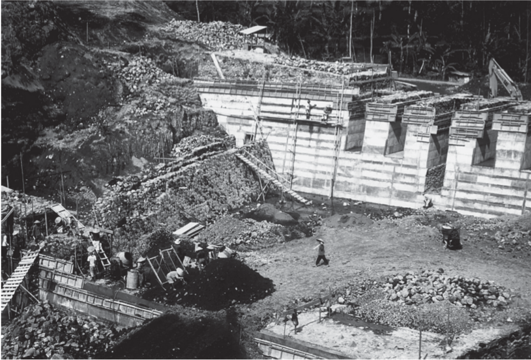
Figure 2.3.2: A sabo dam on the Lamat River, Indonesia, during construction in 1994. Sabo dams are used to impede a natural granular flow, hence reducing its destructive capability. Originally presented by Lavigne et al. [2000].
