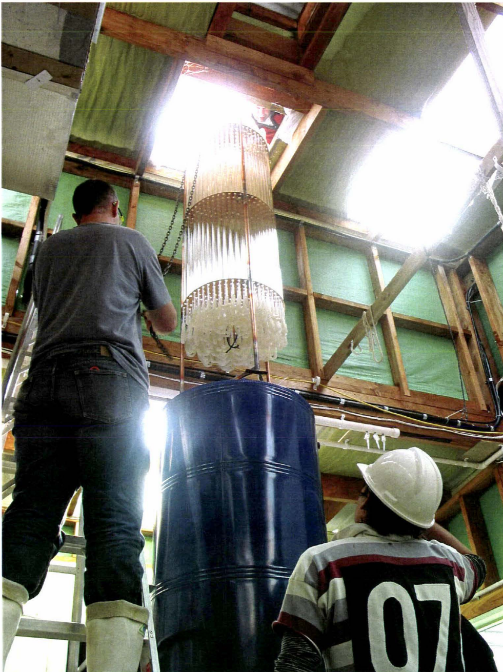
Figure 24 - The copper stand system being lowered into the HWC.
