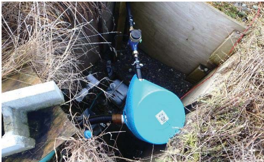
Figure 4.7. Submersible pump in use at the field site for the 2015 drainage season.
