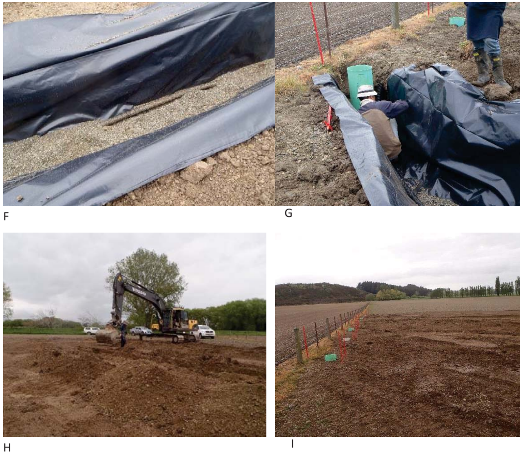
Figure 4.3. Photos of the establishment of the Otama channel lysimeters, November 2012. Photos are: A. Measurement of channel location, B & C. Excavation of channels, D. Lysimeter channel, E, Measuring fall in channel, F. Plastic liner with drainage pipe and pea gravel, G. Connecting drainage pipe to collection chamber, H. Filling in channel lysimeters, I. Site after completion with drainage chambers visible.
