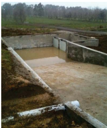
Figure 3.1. Telford barn and effluent system. A. Telford wintering barn and feeding alley, B. purpose-built collection pond and C. small weeping wall in collection pond with wider than normal slats.
