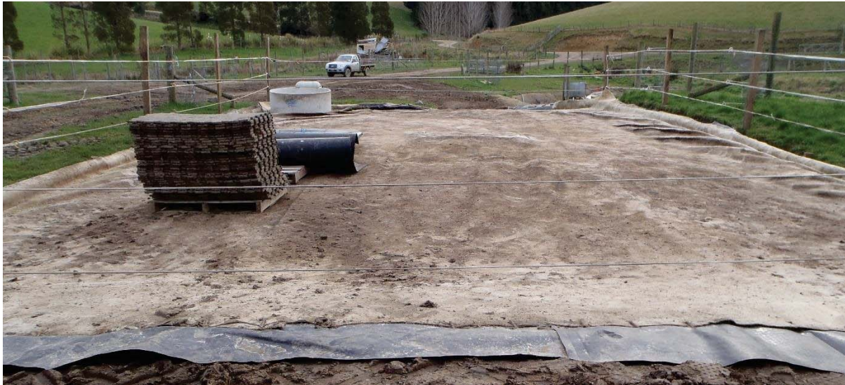
Figure 5.5. Portable pad showing side bunding and electric fence (Kura matting is shown stacked on the left of the photo).
