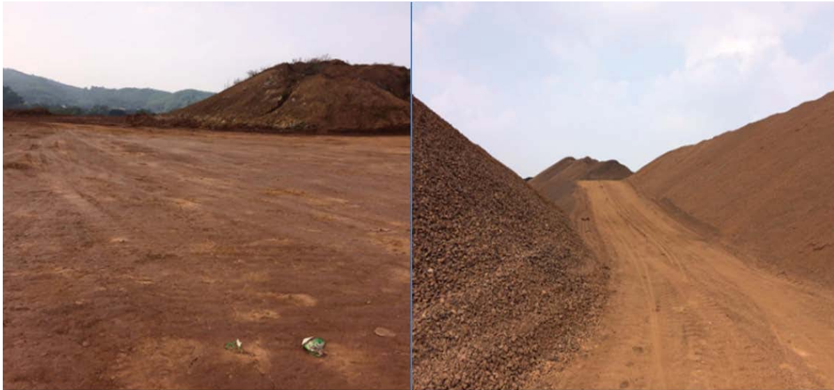
Land clearance for construction
