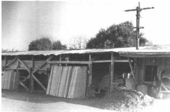
Figure 43 Concrete works at rear of housing, Church Street.
