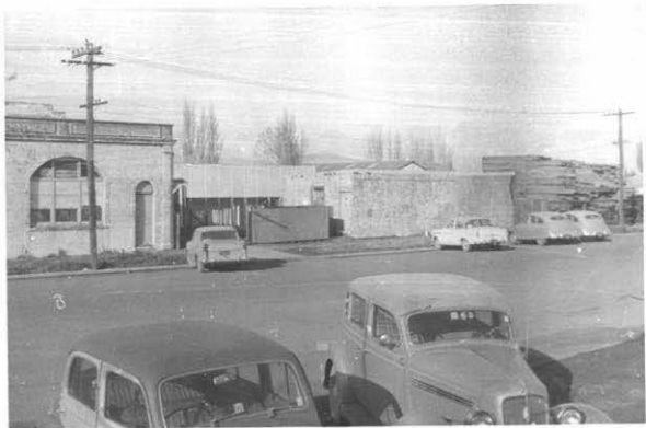
Figure 39 Plaster works and timber yards, Church Street.
