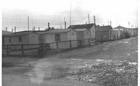
Figure 27 Main St. A disgrace to the Government and an embarrassment to the City, this railway workers' compound is shortly to be removed.
