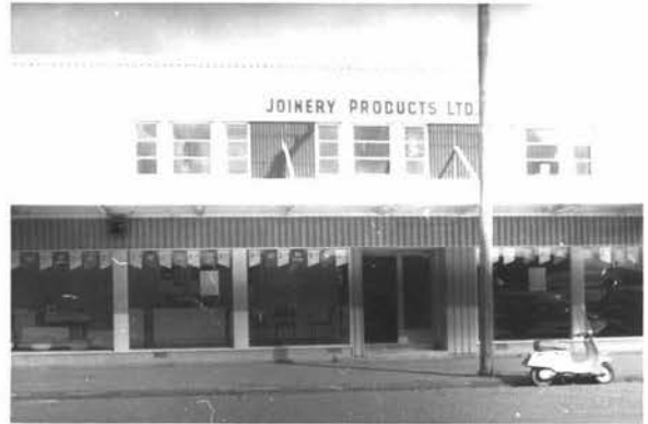
Figure 36 A renovated factory Church Street.
