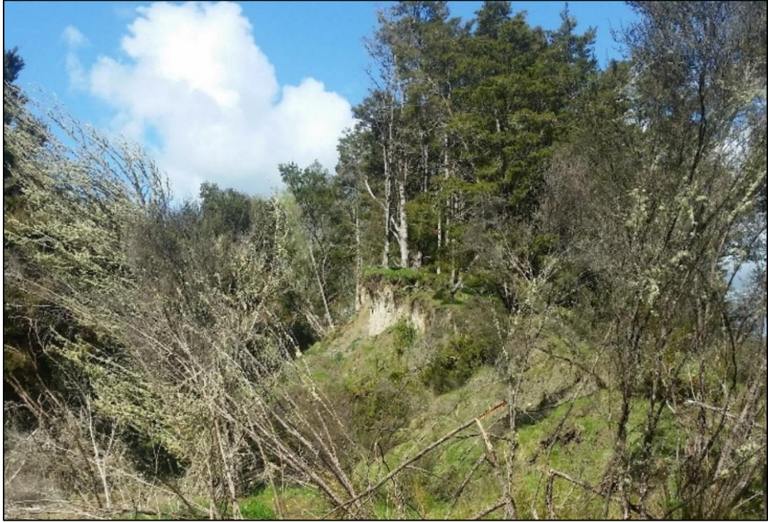
Figure 48. Photo taken in October 2017 from the base of the graben, showing the southern graben edge (position shown in Figure 47).
