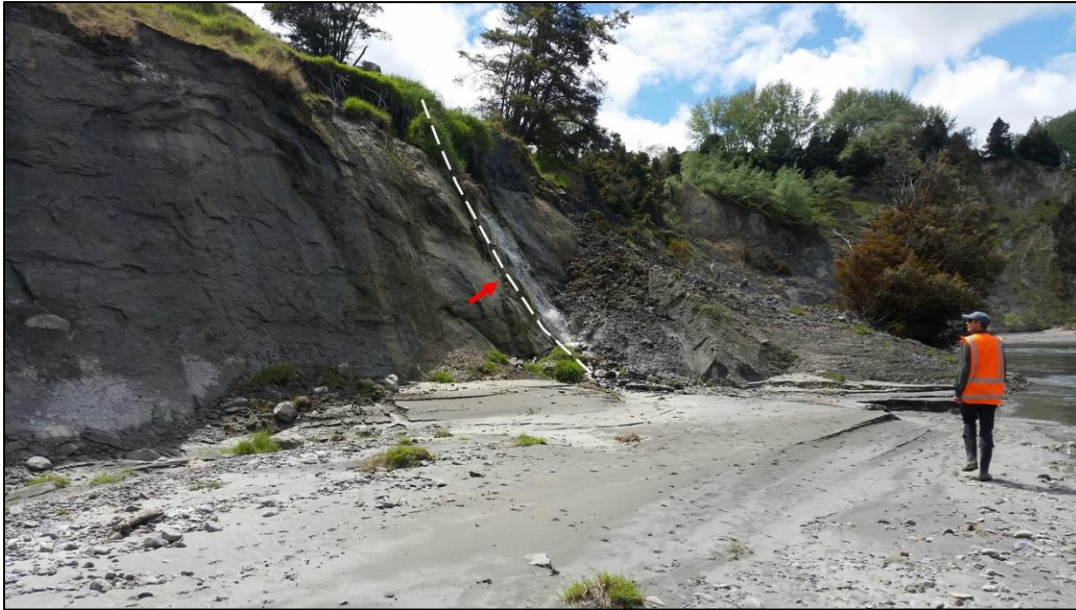
Figure 81. Photograph of the Rangitikei Slide toe front, on the river bank that is not accessible during moderate-high flows. The difference in material behaviour is clear, with the earthflow material to the right and the cohesive bank on the left, and the landslide boundary marked by the stream that flows along the lateral shear (southern-most boundary; shown by the white line and red arrow). The bare-rock cliff is visible to the right.
