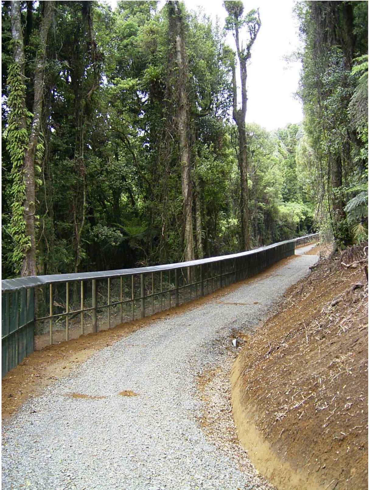
Fig. 2.1- Detail of predator-proof fence along the Maungatautari's Northern Enclosure. Photo by Jillana Robertson
