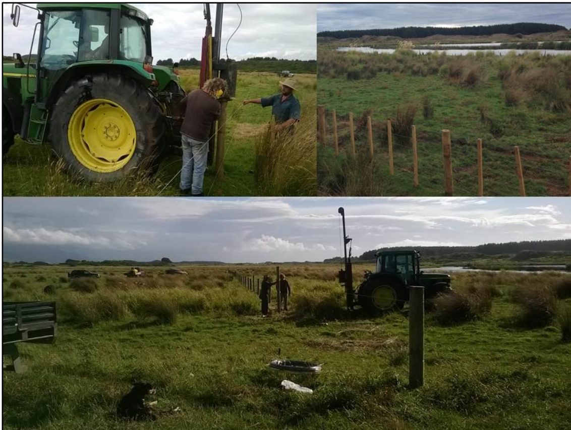
Figure 5.3.2 Fencing in progress at Lake Waiorongomai (Source: top left and bottom photos taken by Rupene Waaka 08 January 2014, top right photo taken by Aroha Spinks 31 March 2014)
