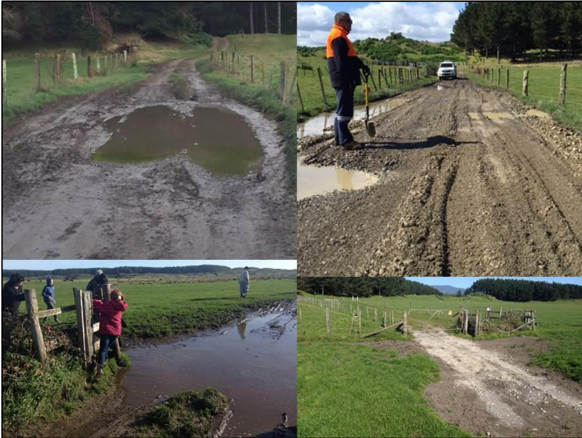
Figure 5.3.19 Before and after gravel was added to the road leading into Lake Waiorongomai and at the entry to Waiorongomai 3B2 (Source: Top photo's taken by Shane Hagai, 11 September 2015, bottom left photo taken by Aroha Spinks, 13 June 2015, bottom right photo taken by Aroha Spinks, 05 October 2015)
