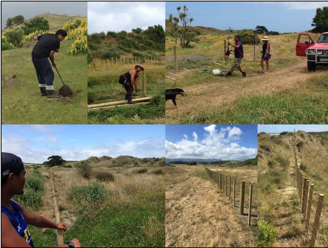
Figure 5.3.12 Fencing of the Waiorongomai Stream (Phase 2) completing the restoration area and padlock on the restoration front gate of the Lake Waiorongomai restoration area. Photo's clockwise from the top left, Meihana Taurima digging initial post holes (Source: photo taken by Aroha Spinks, 11 November 2014), Skip in action fencing alongside photo of Meihana Taurima and Tuihana Nikora-Whiting (Source: photo's taken by Aroha Spinks, 18 January 2015), bottom three photos are of phase 2 fence lines completed (Source: photo's taken by Aroha Spinks, 05 February 2015)
