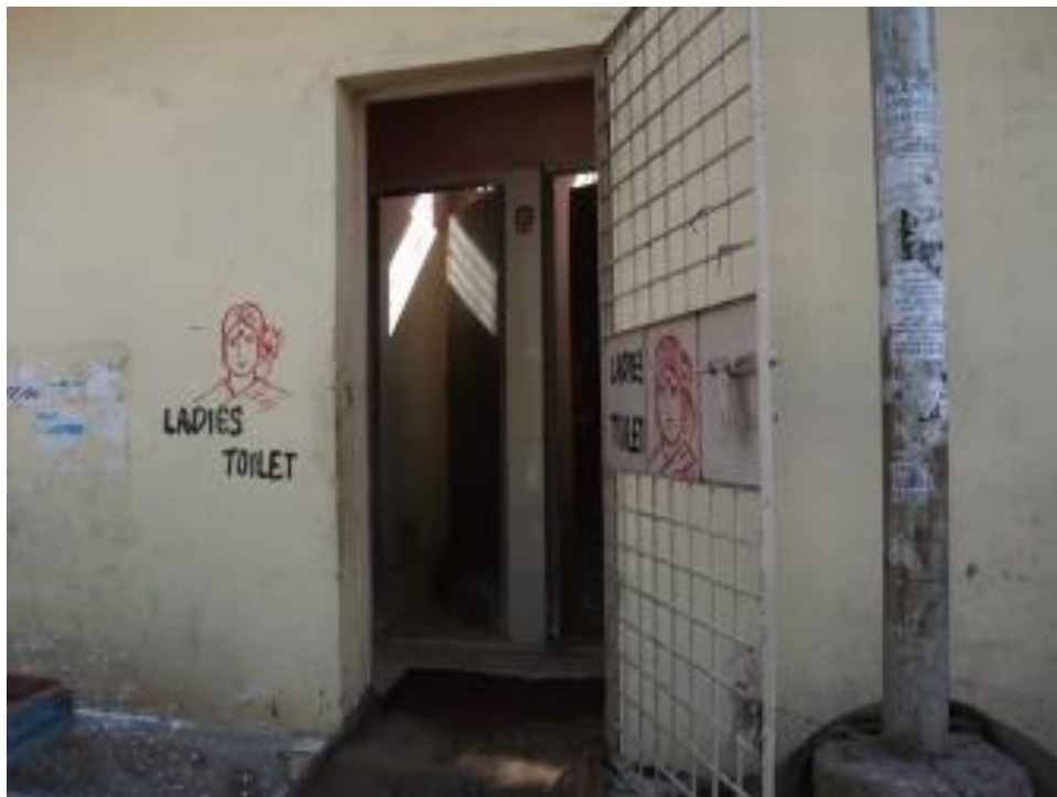
Figure 30: Entrance to women's toilets
