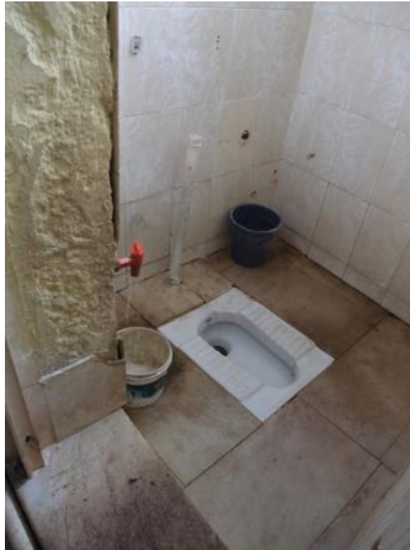
Figure 24: Toilets upstairs at KR Market
