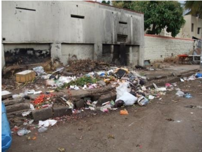
Figure 38: Rubbish pile before
