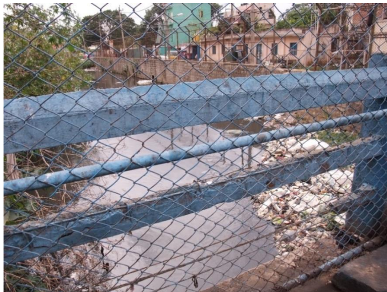
Figure 6: Run off from one of the lakes with rubbish accumulated by the banks
