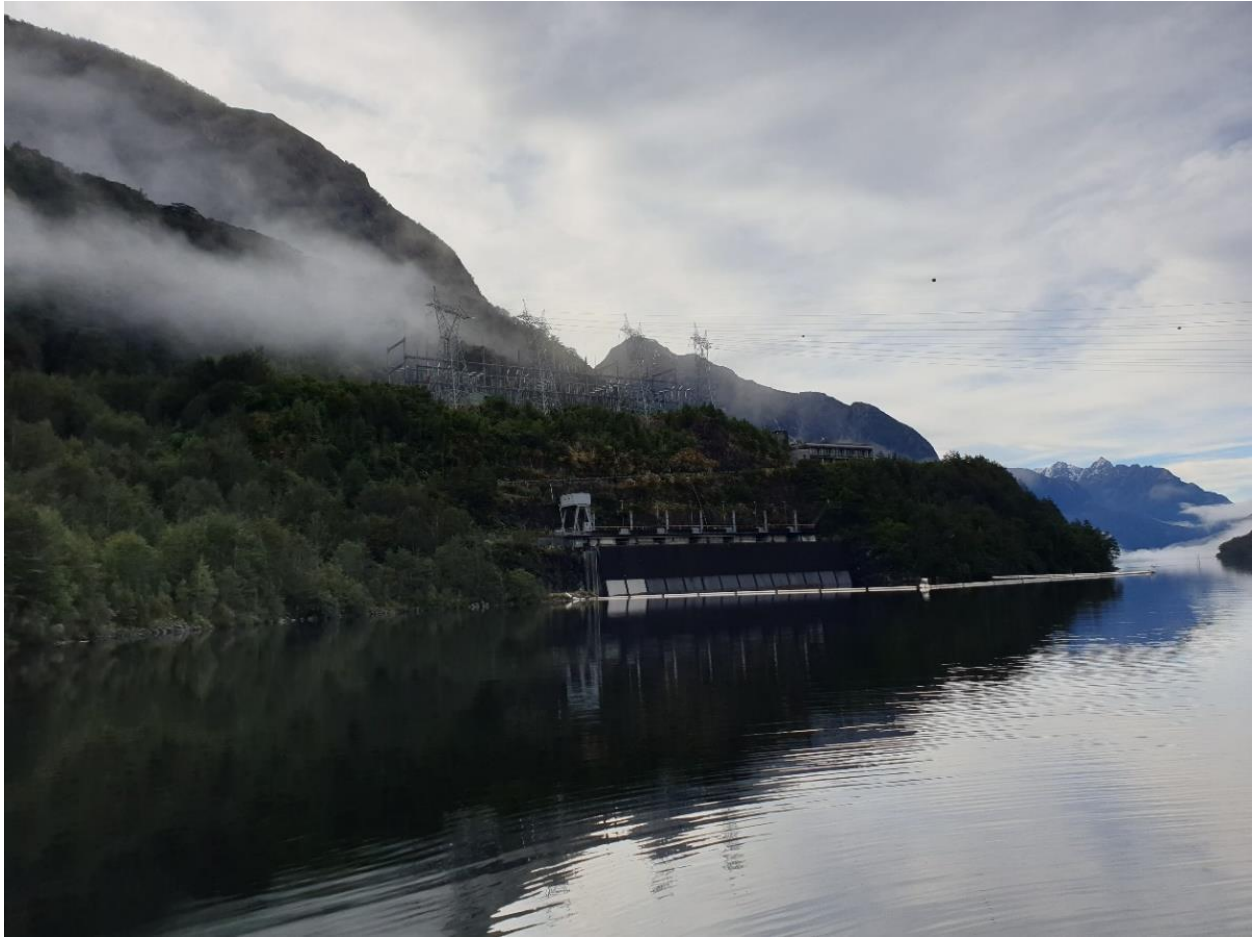
The Manapōuri Power Station at West Arm, Lake Manapōuri (source: Waiau Rivercare Group Inc. (2019)).
