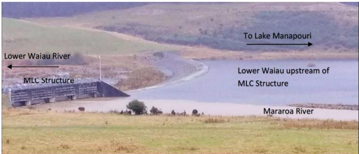
Figure 4: The MLC diverting sediment laden Mararoa waters through the Weir to the lower Waiau River (source: Waiau Rivercare Group Inc. (2019)).
