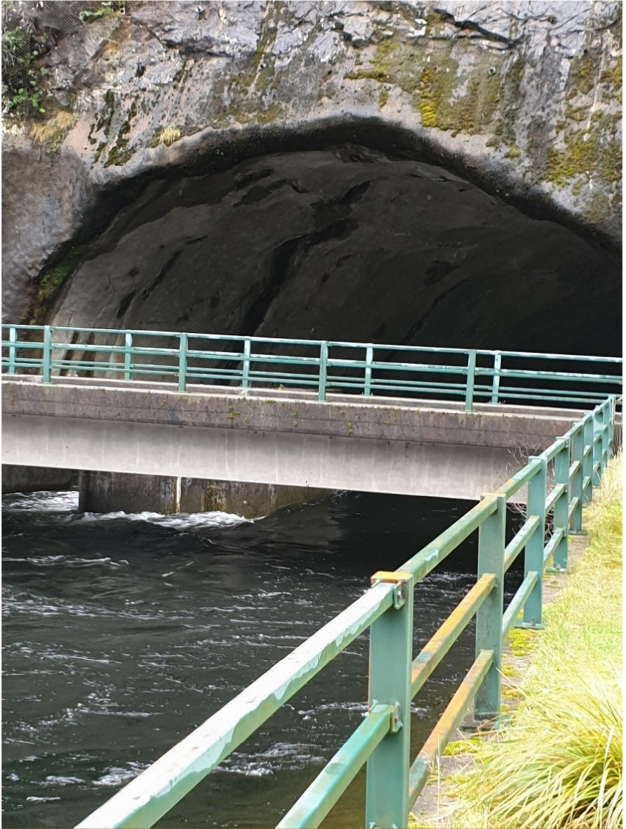
Figure 5: Waiiau River water exiting one of two discharge tunnels at Deep Cove, Doubtful Sound (source: Waiiau Rivercare Group Inc. (2019)).
