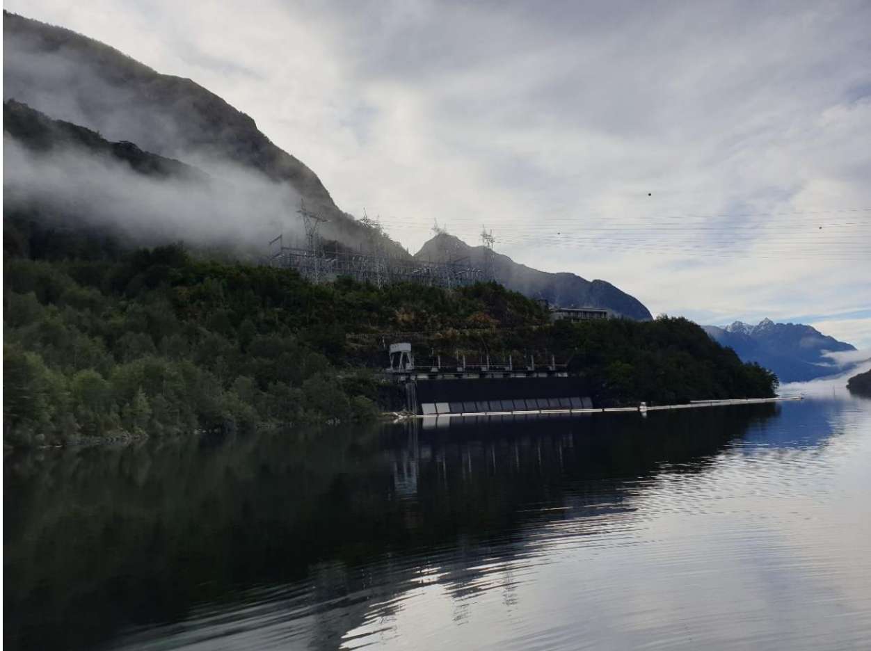
Figure 6: The Manapōuri Power Station at West Arm, Lake Manapōuri (source: Waiau Rivercare Group Inc. (2019)).
