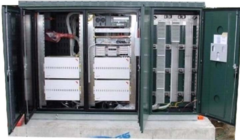
Figure 5.14: ISAM in a roadside cabinet
