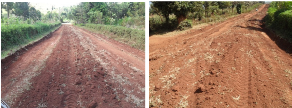
Figure 13 State of the road between Nchiiri to Kagaene while they were being graded
