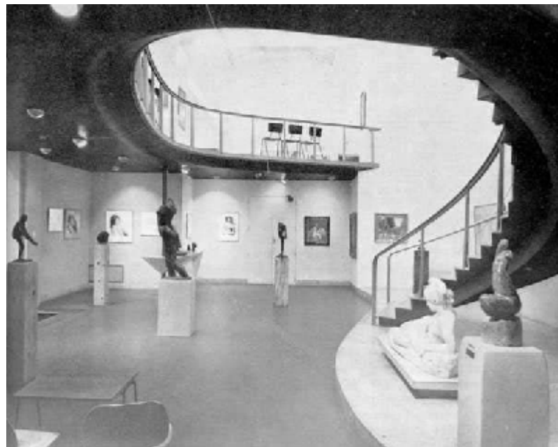
Plate 3.6 New Sculpture Court, Auckland City Art Gallery, 1950s. This area was created by inserting a mezzanine into the Mackelvie Gallery. The contrast between this photograph and that above is an indication of the changes introduced by Westbrook.
