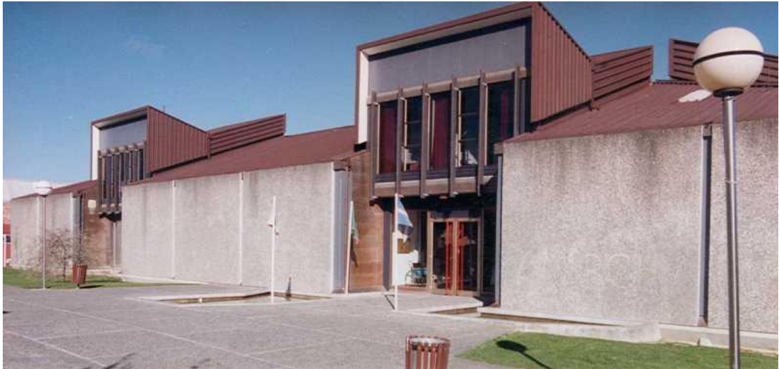
Plate 5.9 Exterior of the new Manawatu Art Gallery building on Main Street, 1988.
