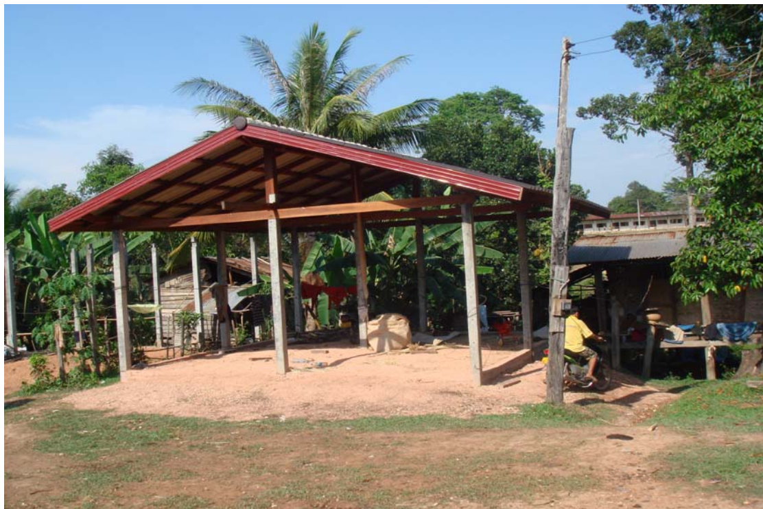
Figure 5.3: A farmer's new house under construction after 4 years of working in the project.
