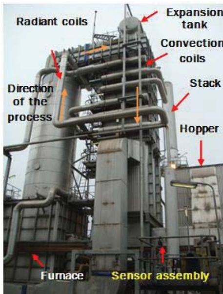
Figure 35: Far view of carbon monoxide/oxygen analyser Located at the plant (heating plant 1)
