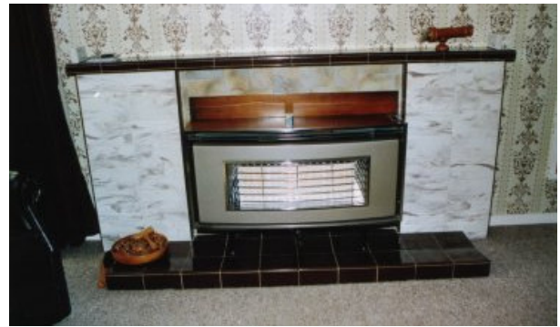
Figure 5.6 Reticulated gas heater
