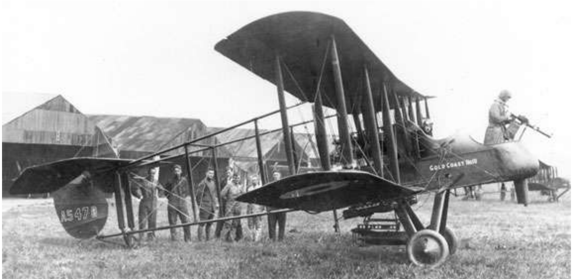
Figure 6: F.E.2 , one of the RFC's answers to the Fokker Eindecker in a 'pusher'-type configuration. The F.E. 2 was a two-seater multi-role aircraft, with the gunner located at the front of the nacelle. Source: www.theaerodrome.com
