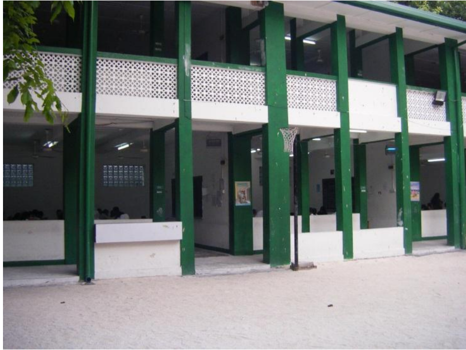
Figure 10: Classrooms with half open walls.
