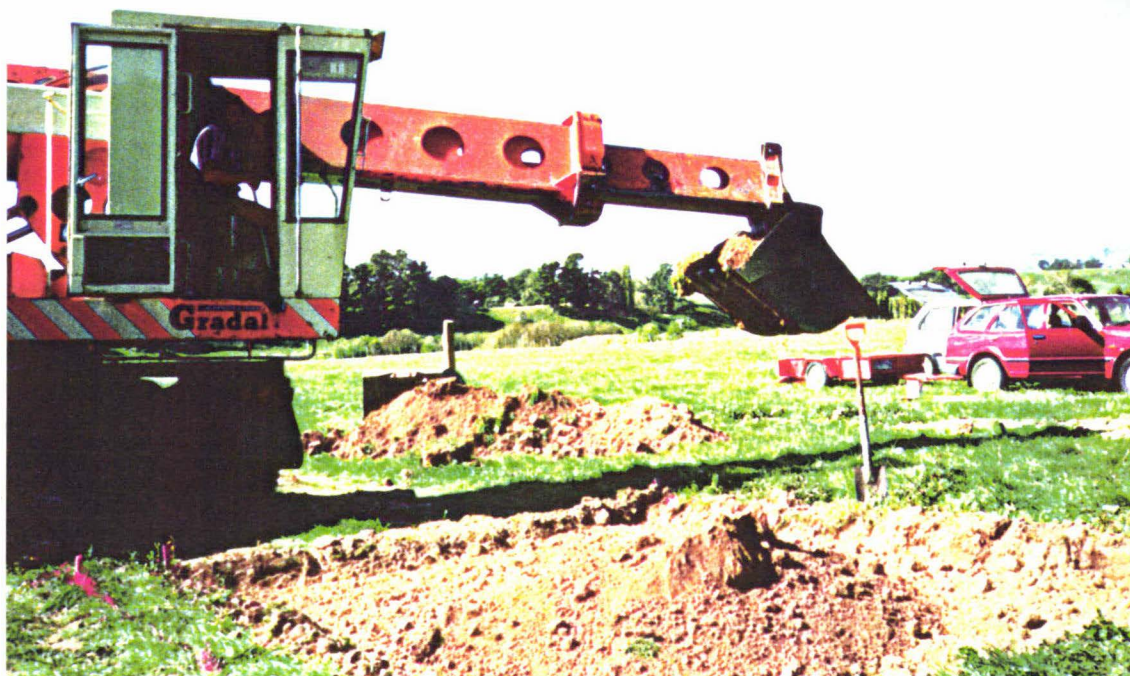
Photograph 4.6: Construction of the Ohakea trial: The darker A horizon is being replaced on top of the lighter B horizon of an "AonB" treatment.
