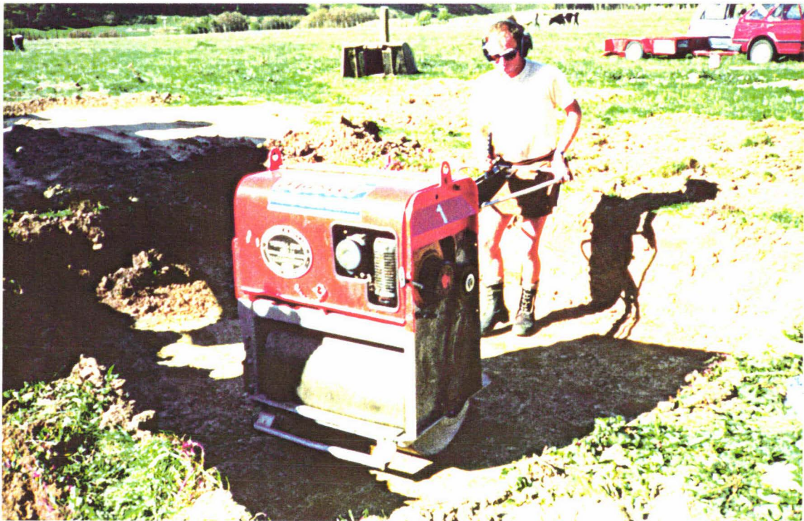
Photograph 4.7: Ohakea trial construction. The base (c.0.5 m deep) of an "Aonly" treatment is being compacted with a vibrating roller.
