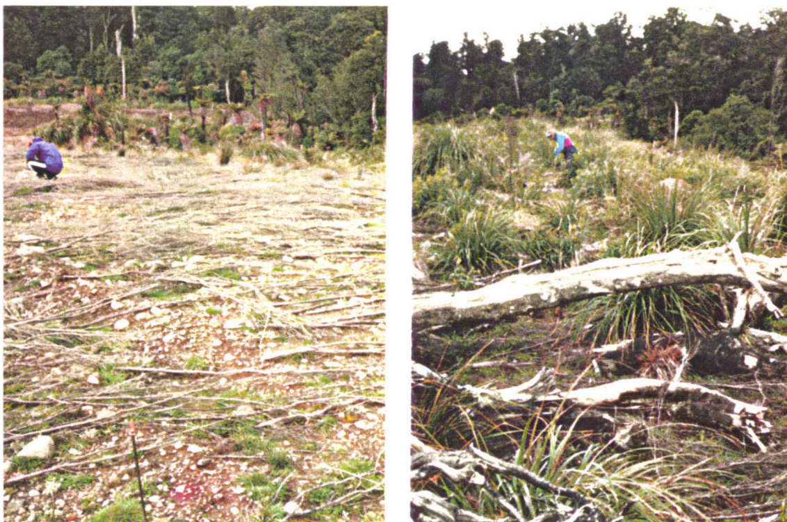
Photograph 3.6: Reclamation of a stockpile of laharic material adjacent to the main trunk railway, Ohakune. Manuka slash was either laid directly on the laharic material (LHS) or on a 0.3 to 0.5 m layer of replaced forest soil (RHS).
