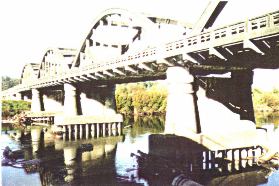
Photograph 2.4: Exposed pilings of the old Fitzherbert Bridge over the Manawatu River, Palmerston North in 1987, due to unsustainable extraction of aggregate from the river.
