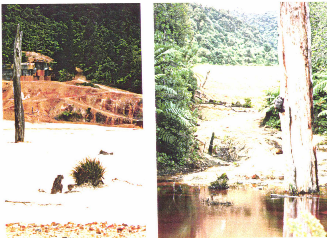
Photograph 3.4: The tailings pond, battery (LHS) and tailings pond bund above the sediment settling pond which contains toxic rust-coloured leachate (RHS) at the Tui mine. Vegetation only grows on "islands" of organic matter on both ponds.
