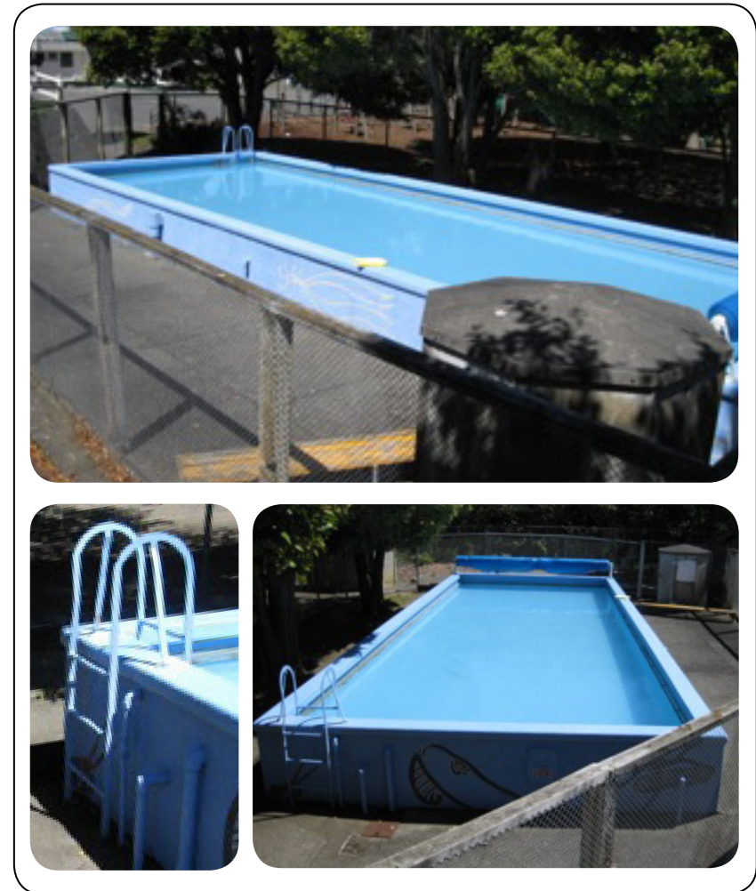
Figure 11. The traditional Reid Pool with single steel ladder entry. Te Aro School, Wellington, NZ.
