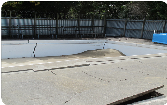
Figure 72. The swimming pool at Beckenham School in Christchurch damaged by the earthquake on the 22 February 2011.
