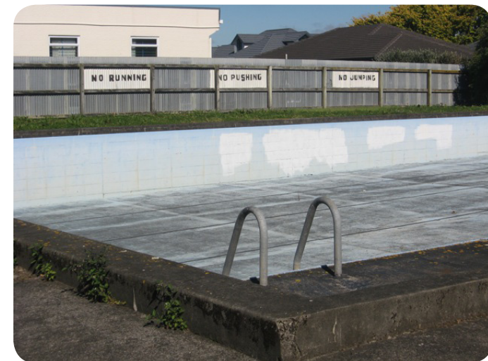
Figure 1. Decommissioned pool, Avalon Intermediate, Lower Hutt NZ.
