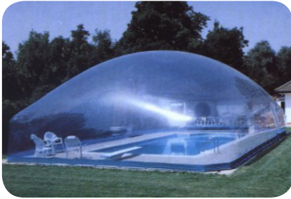
Figure 44. Single layer pressurised pool enclosure.
