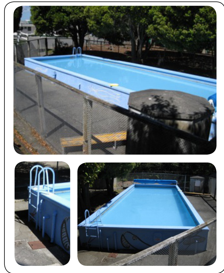
Figure 83. The traditional Reid Pool with single steel ladder entry. Te Aro School, Wellington NZ.
