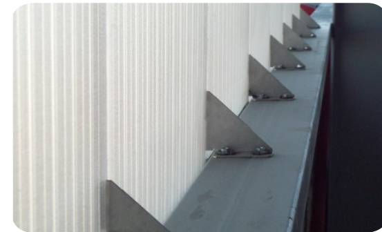
Internal metal fasteners hold the sheets onto the steel purlin.
