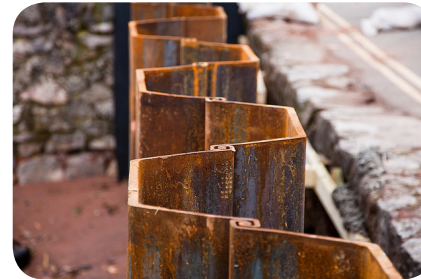
Figure 98. A sheet piling wall combines a strong structure with the ability of the components to nest together.
