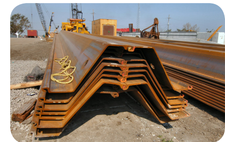
Figure 98. A sheet piling wall combines a strong structure with the ability of the components to nest together.
