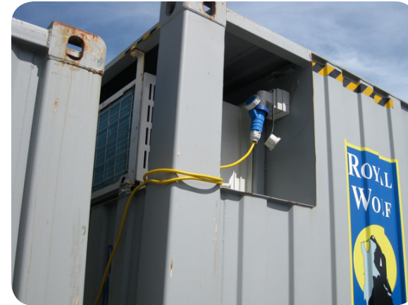
Figure 70. A single phase power inlet on a modified shipping container.
