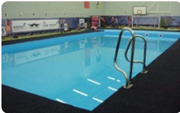
Figure 22. Pools 4 Schools pool. The raised platform around the pool creates an 'in-ground' pool experience.
