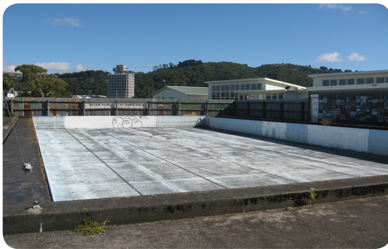
Figure 7. Decommissioned pool, Avalon Intermediate School, Lower Hutt, NZ.
