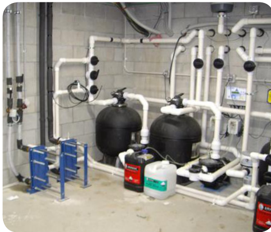
Figure 26. A swimming pool plant room.
