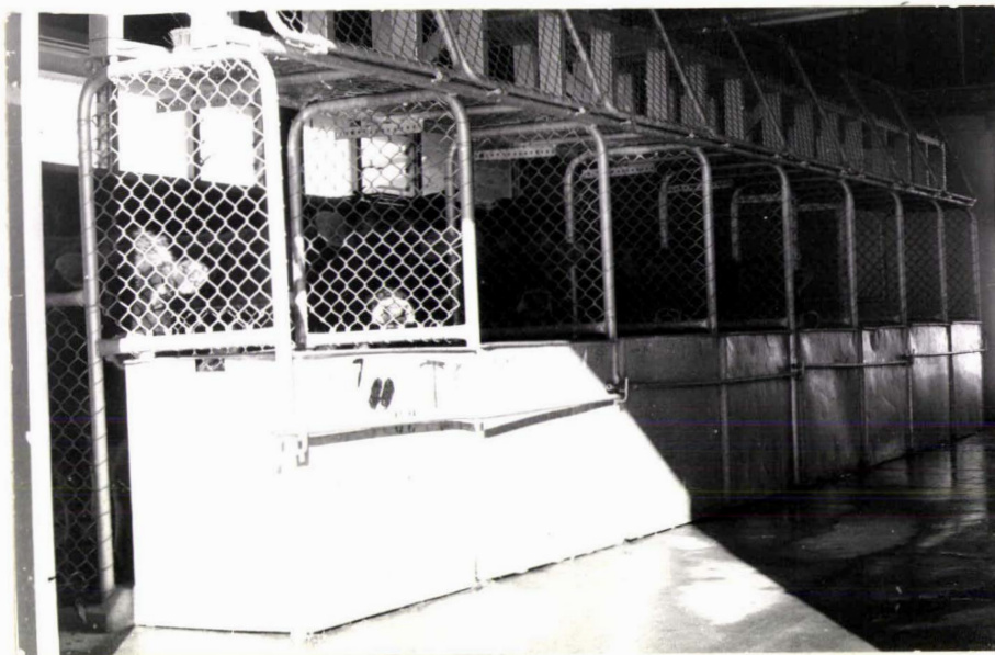
PLATE 2: Interior of the Feeding Barn
