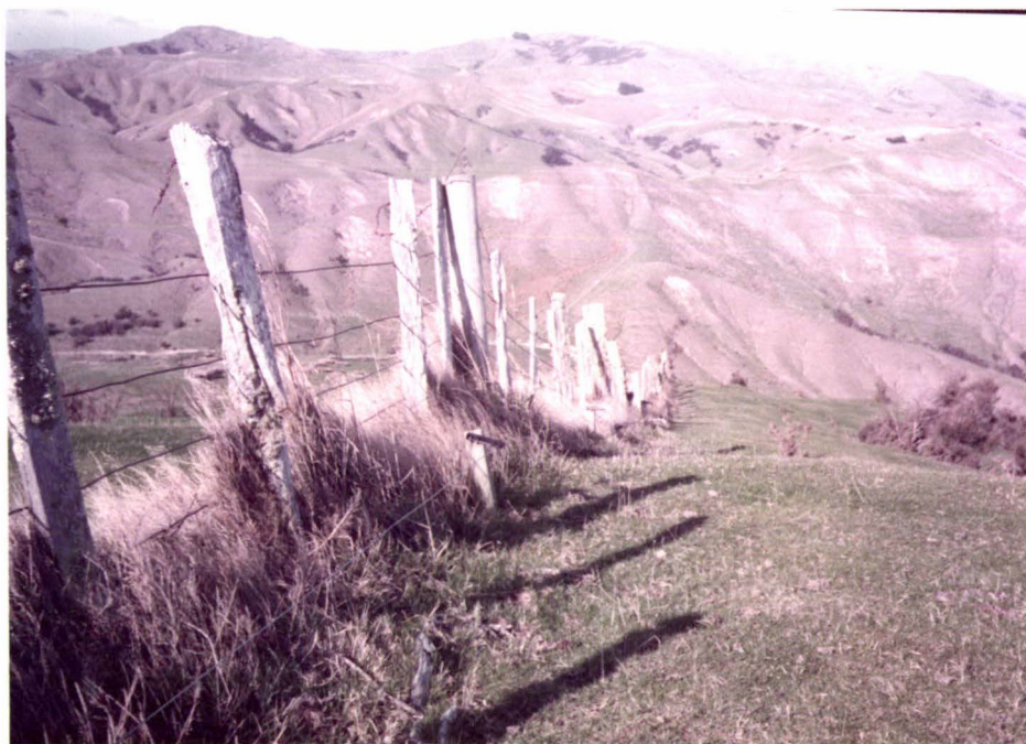
Plate 3.2 Erosion during September 1977 is still clearly visible in southern Bideford. Note the use of electric outrigger to stock-proof old conventional fence.
