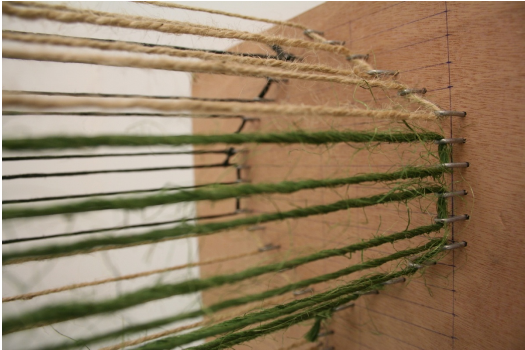
Figure 5.14. Detail of installation showing the fibrous nature of the lashing and zinc staples.
