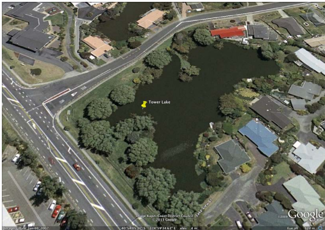
Figure 14. Tower Lake No 1 on the corner of Langdale Avenue and Kapiti Road.
