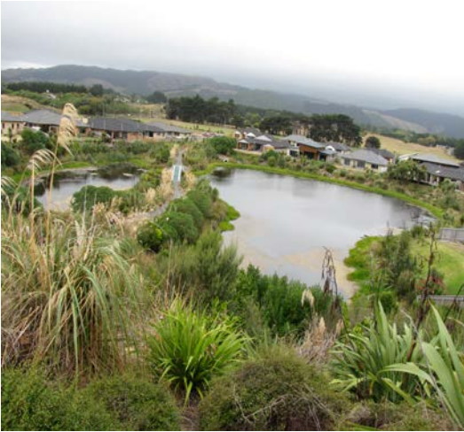
Figure 19. Lake Kotuku stormwater collection pond south arm from adjacent constructed sand dune. (Photo: K. Palmer 2010).
