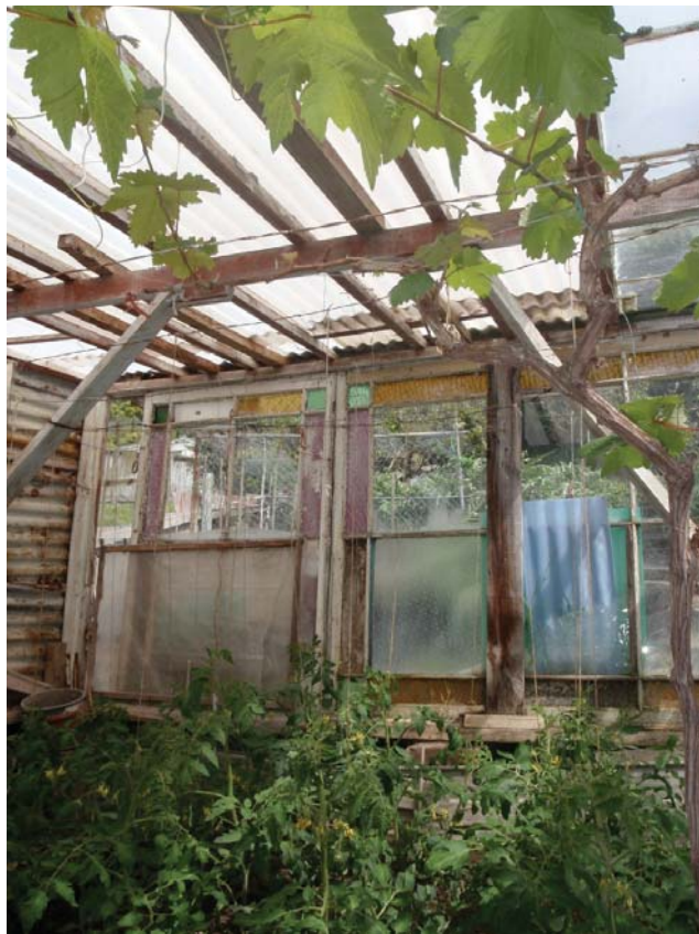
Figure 13. A glasshouse built from recycled materials, with tomato plants and grapes.
