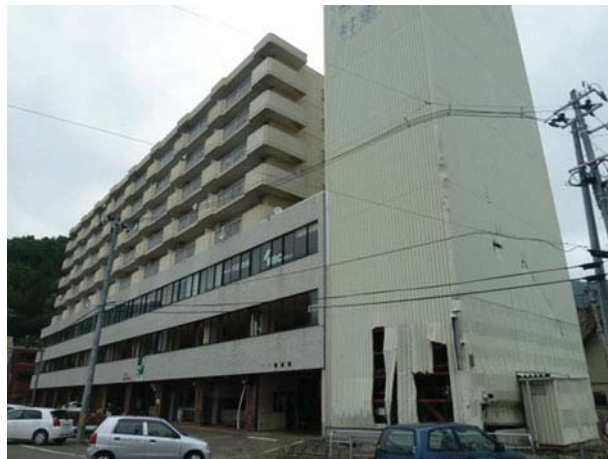
Fig. 6 Eight storey un-braced RC shear wall apartment block and designated evacuation building in Kamaishi City. A steel frame structure is located on the seaward face and sustained minor damage from debris impact. Two external staircases to the 4th floor exist on the other side of the building. This building was inundated to the 3rd storey
