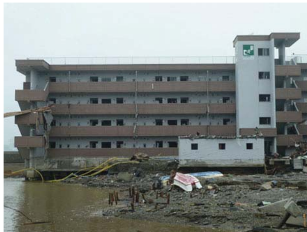
Fig. 13 The Matsubara apartment block and designated vertical evacuation building in Minami-Sanriku. This photograph shows the landward side of the building with scour of at least 2 m at its northern end (a similar amount of scour was also observed at the southern end). Observations of this side of the building show little structural damage despite 16 m inundation height
