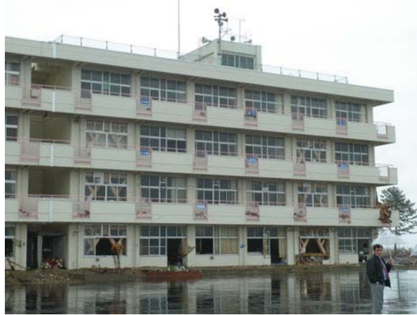
Fig. 22 The south side of Arahama Elementary School, which was successfully used for vertical evacuation. Timber-clad steel bracing is visible in windows of the lower floors. Damage to non-structural components at the ground floor is shown, along with debris at the seaward end of the building on the second floor. The roof shows evacuation infrastructure including warning sirens and fencing around an evacuation area. There is external access to the roof on the north side of this building
