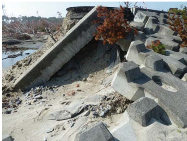
Fig. 21 Failure of a concrete block revetment at Arahama Beach. Sand fill had been washed out of the revetment, causing collapse of the concrete blocks and pathway along the crest of the defence
