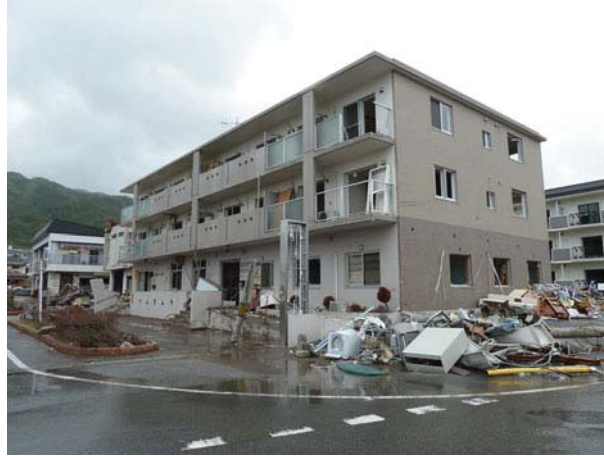
Fig. 7 Apartment building of RC shear wall construction in Ōfunato City. Seaward side of the building is shown. Inundation reached the ceiling of the 3rd floor, but the structure remained intact. This landward side of the building was sheltered from debris impact during the tsunami return flow
