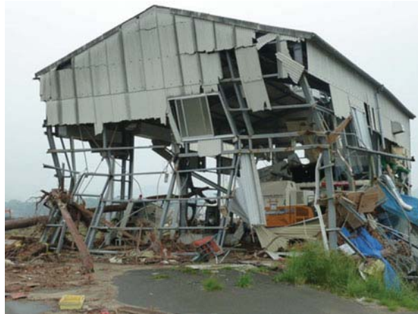
Fig. 25 A steel frame agricultural building located 1 km inland at Yamamoto Town, Miyagi Prefecture. A tree trunk, apparently from the damaged coastal pine forest, struck a structural column on the south-east (seaward) corner of the building, buckling the structural and non-structural members. Tsunami flow has removed cladding to a height of over 4 m
