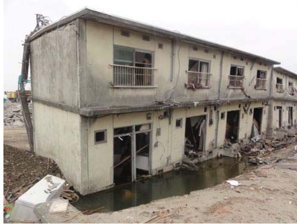
Fig. 24 View along the north side of one apartment block in Yuriage, illustrating scour at the seaward end of one apartment building. Loss of soil providing bearing capacity to support the footings resulted in tilting of this building
