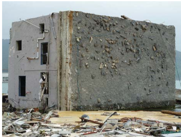
Fig. 18 An overturned two-storey RC shear wall structure with raft foundations at the harbour edge in Onagawa Town—'Building B'
