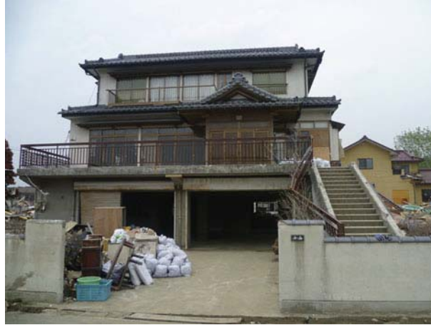
Fig. 9 An example of a timber frame dwelling constructed with an RC ground floor structure. The main house is 3 m above ground level, 780 m inland and 60 m from the river. Despite inundation depth of approximately 6 m in this area, the house had sustained very little non-structural damage
