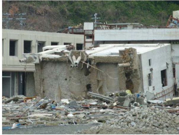
Fig. 17 Foundations of an overturned two-storey RC shear wall structure with piled foundations in Onagawa Town—'Building A'. Evidence of impact at the roof of the building on its seaward side indicates that this failure may have been initiated by debris strike
