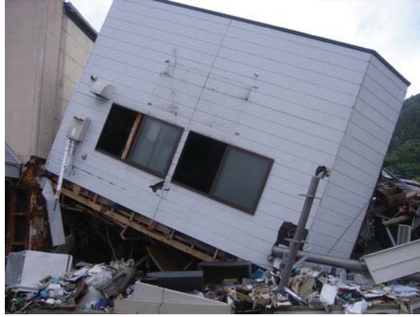
Fig. 5 Soft storey collapse of a timber structure observed in Kamaishi City. The 2nd storey appears to have remained intact due to central steel beam supporting the second storey
