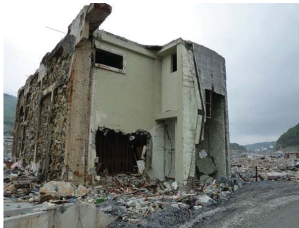
Fig. 20 A 2-storey RC shear wall structure with shallow pad footing foundation ('Building E'). Evidence of small piles on at least one of the corner columns can be seen, but no piles remained attached at the time of our visit. The building has also sustained out-of-plane failure of an infill wall at the ground floor
