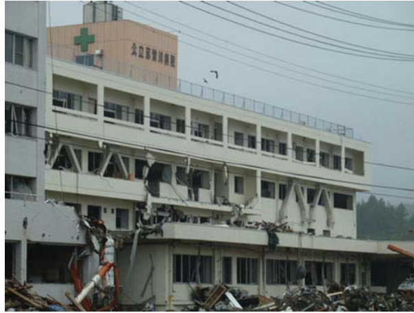
Fig. 14 Shizugawa Hospital, Minami-Sanriku, which was inundated to 11 m depth but was used in evacuation to the roof. This photograph shows the landward side of the building with evidence of damage to the balcony at the 4th storey
