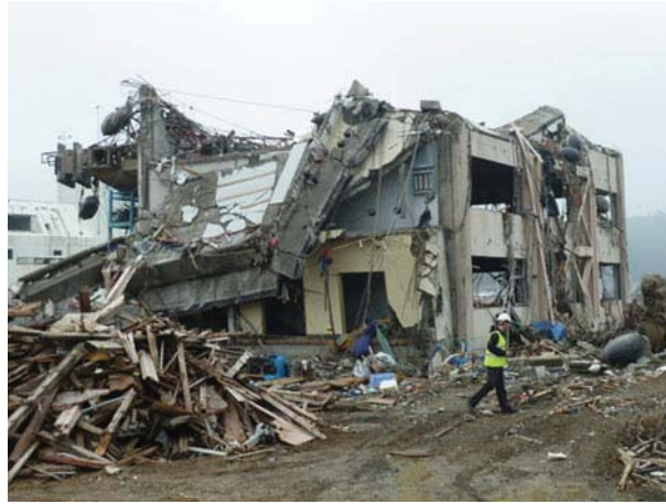
Fig. 12 RC building in Shiomi-cho, Minami-Sanriku, 100 m from the sea ( 38^{\circ} 40' 29.10'' N, 141^{\circ} 26' 44.96'' E) showing collapse of upper storeys. Several other RC buildings in the immediate vicinity of this building had suffered collapse with evidence of severe scour and debris impact
