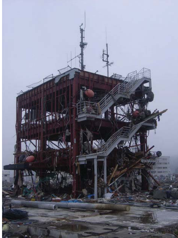
Fig. 11 The 3-storey steel frame Crisis Management Department (CMD) building, located 470 m from the harbour front. This building was inundated to the roof (at 10 m elevation above ground level) and sustained loss of all cladding although the structure remains standing. Damage to this building and the deaths of CMD staff resulted in the loss of crisis management facilities and expertise in the immediate aftermath of the tsunami
