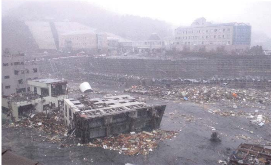
Fig. 19 An overturned 3-storey steel frame building ('Building D') on piled RC foundation with evidence of debris impact on the (originally) seaward face of the building. This photograph was taken from a neighbouring building during tsunami inundation, courtesy of Miyagi Prefectural Office
