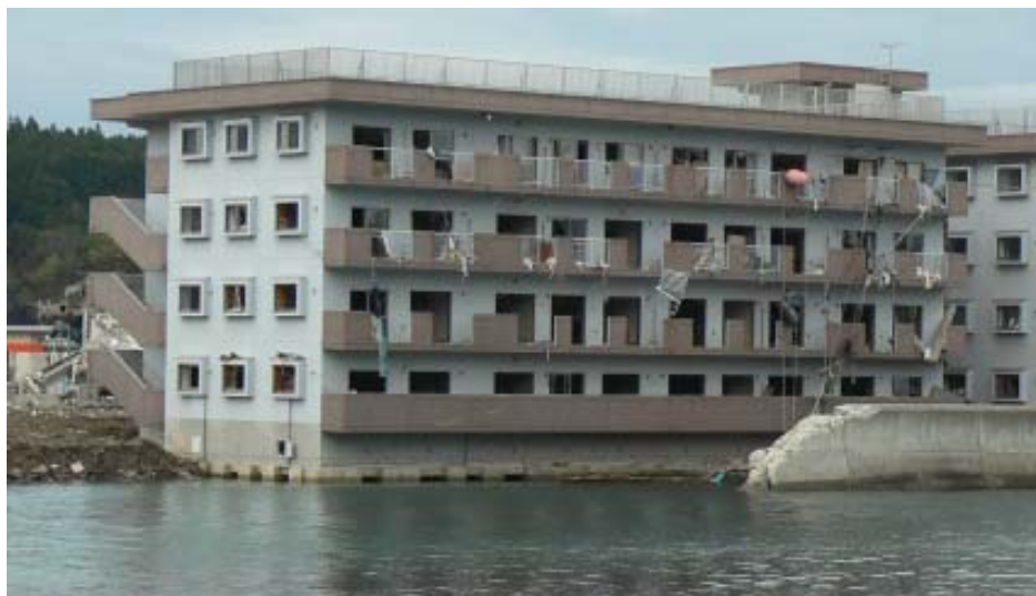
Figure 55 Matsubara apartment block viewed from the seaward side with waterborne debris to the 4 th storey. The low seawall has been destroyed in the tsunami return flow and was sheltered in part by the apartment building. The foundations of this building are exposed above the water level due to extensive scour.
