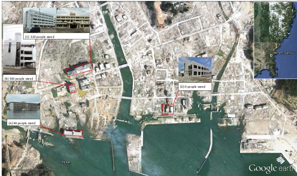
Figure 54 Locations of designated tsunami evacuation buildings in Minami-Sanriku Town: (A) Matsubara apartments; (B) Takano Kaikan building; (C) Shizugawa Hospital; (D) Fisheries Co-operative. Significant scour can be seen where seawater is encroaching around building (A) and to the east of building (D).
