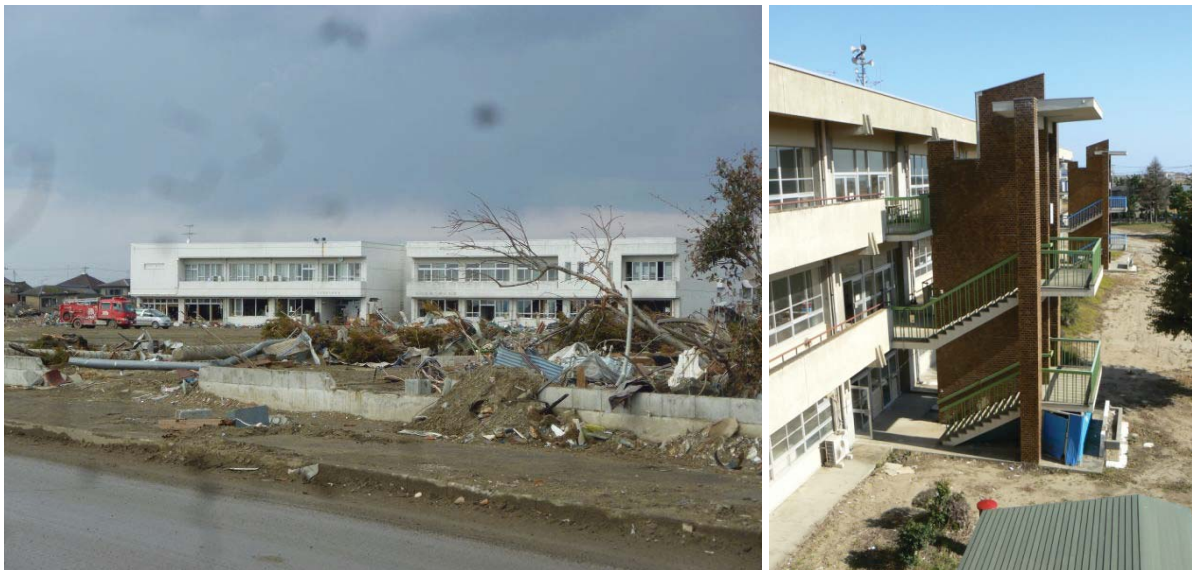
Figure 65 The Yuriage Community Centre was inundated to the 2 nd storey but 43 people survived in the building.
