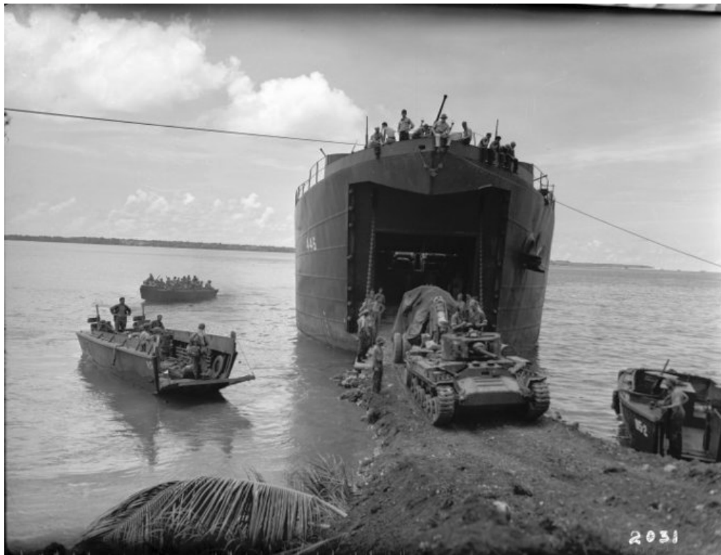
Image 16: 'Getting 'em ashore' – a Valentine tank of the 3 rd NZ Division (towing a US 90mm anti-aircraft gun) drives off an LST onto a coral and earth-made pier constructed by New Zealand engineers, 15 February 1944. (Source: "World War II vehicles, equipment, and troops landing on Nissan Island, Papua New Guinea", New Zealand, Department of Internal Affairs, War History Branch: Photographs relating to World War 1914-1918, World War 1939-1945, occupation of Japan, Korean War, and Malayan Emergency, Ref: 1/2-044755-F, Alexander Turnbull Library, Wellington, New Zealand, http://natlib.govt.nz/records/22720410 .)
