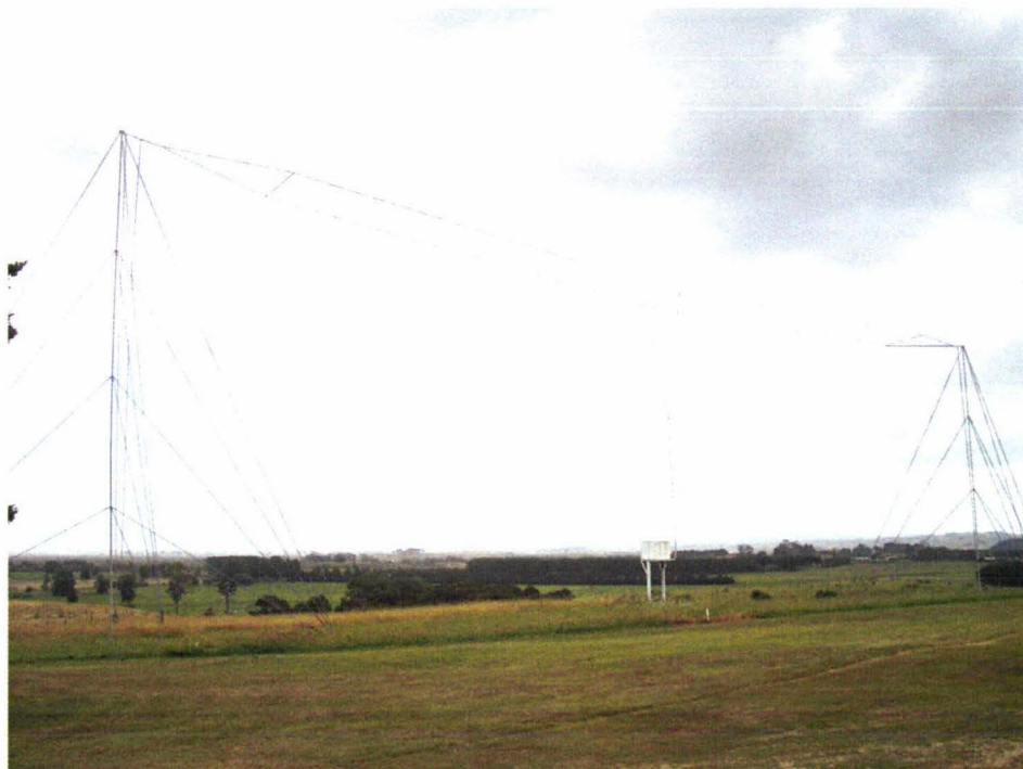
Figure 14. The Surrey NDB Ground Station Transmitter.
