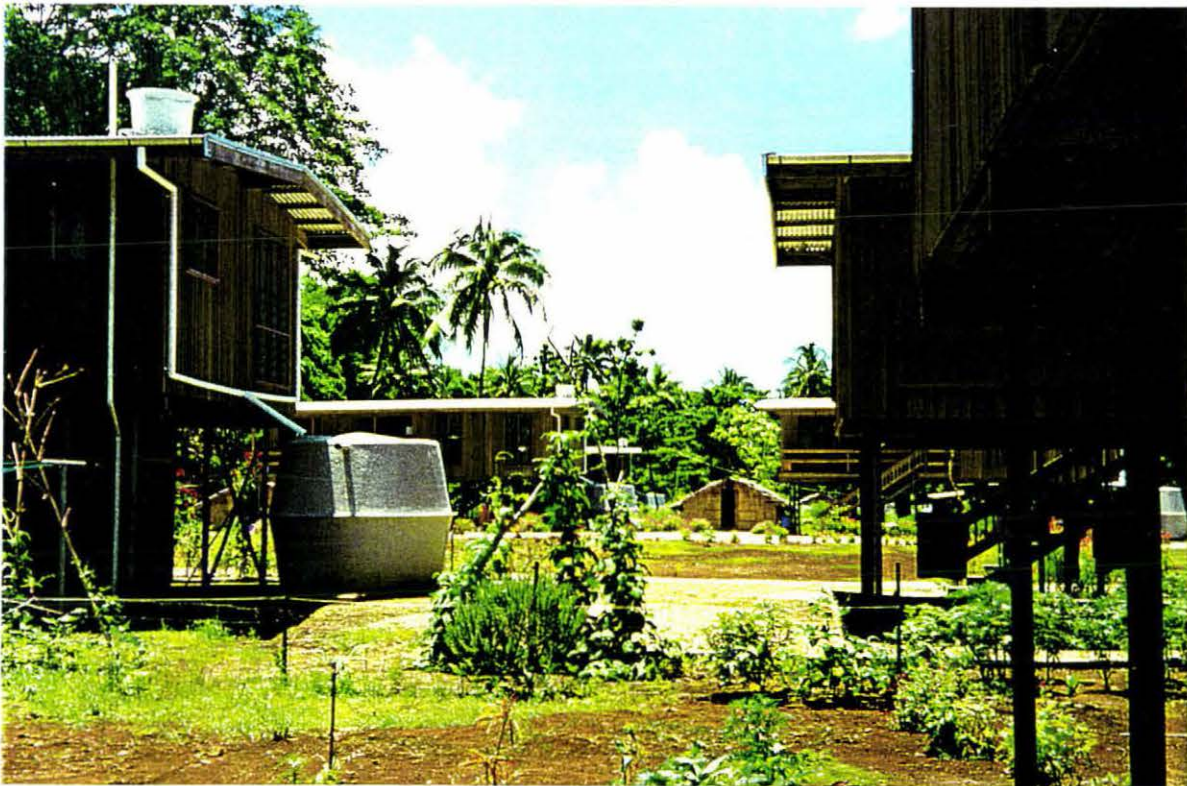
Photo 14: Part of the new Putput 1 village settlement. The displaced villagers are compensated with fully furnished company built houses.
