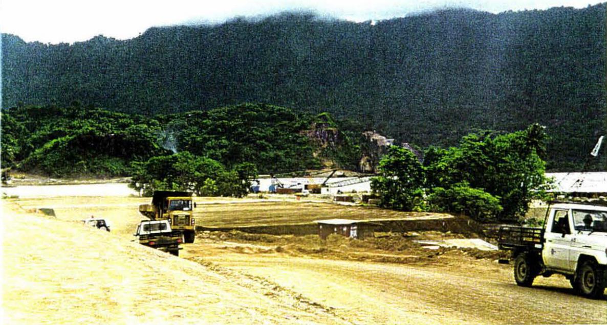
Photo 13: Earthworks and building construction at the Putput plant site. This area was once Putput 1 village. Putput 1 villagers have since been relocated to a new village site.
