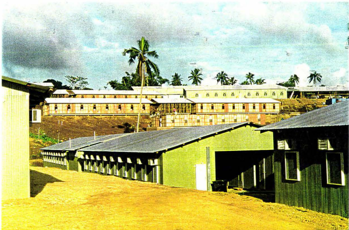
Photo 12: As part of rapid infrastructure development, building and site construction are currently in progress. This is part of the mining camp where LMC and associated company employees are living.
