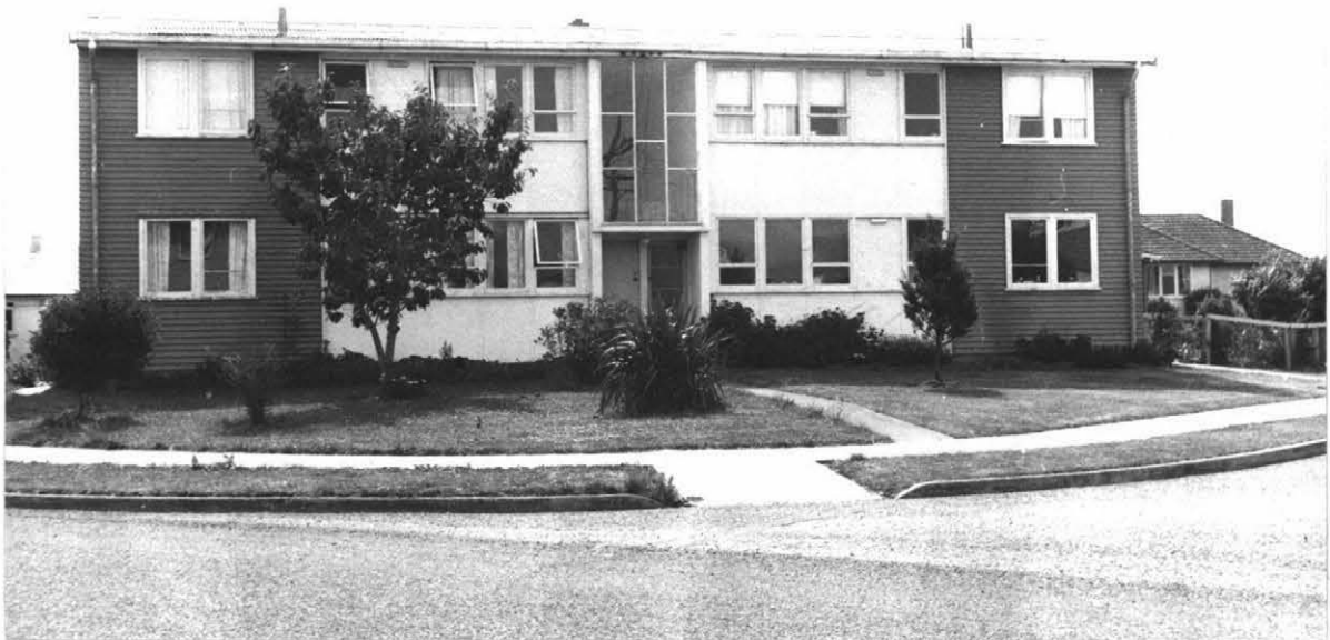
Figure 12. Two-Storey Four-Unit Flats, Hull Place. There are four such buildings in Takaro, each containing two ground-floor and two first-floor flat units.
