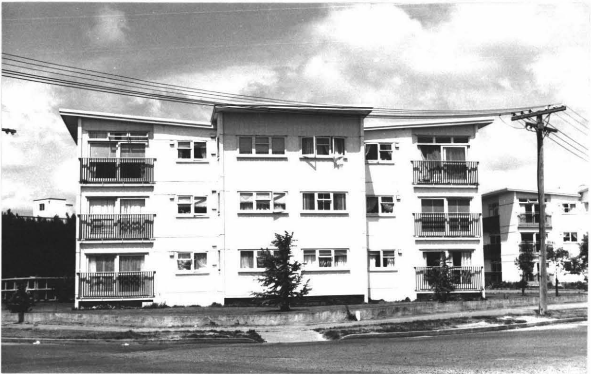
Figure 11. 'Star' Flat, Botanical Road. One of the two 'Star' Flats in Takaro. These three-storey concrete buildings contain twelve flat units.
