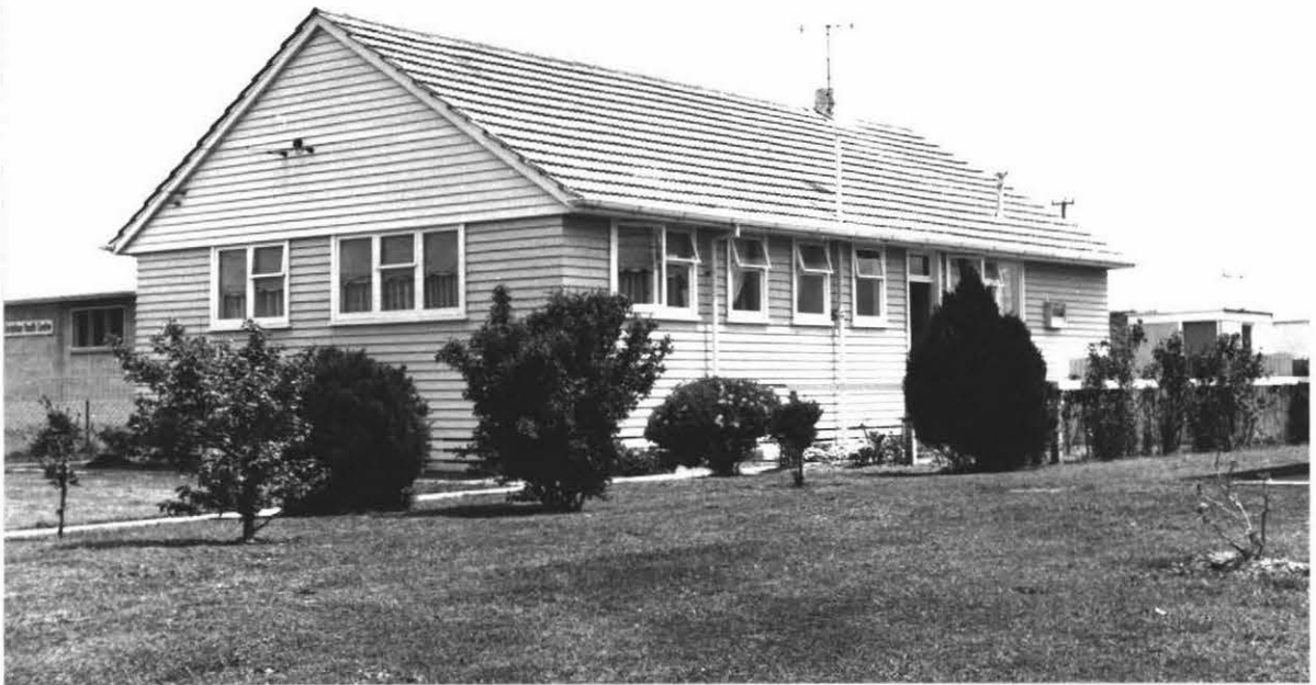
Figure 17. Detached State House, Coventry Street. A typical detached house.
