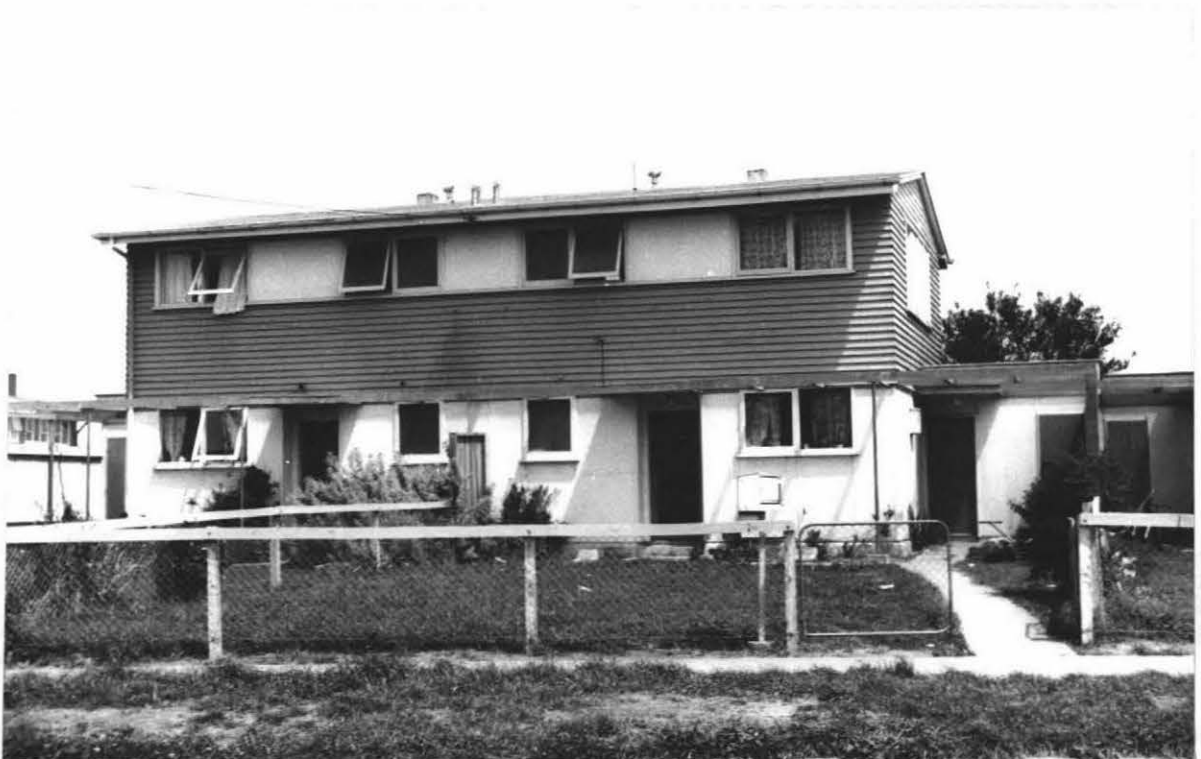
Figure 14. Two-Storey Double-Unit, Botanical Road. The dilapidated condition is typical of a small, but noteworthy number, of similar buildings in Takaro.
