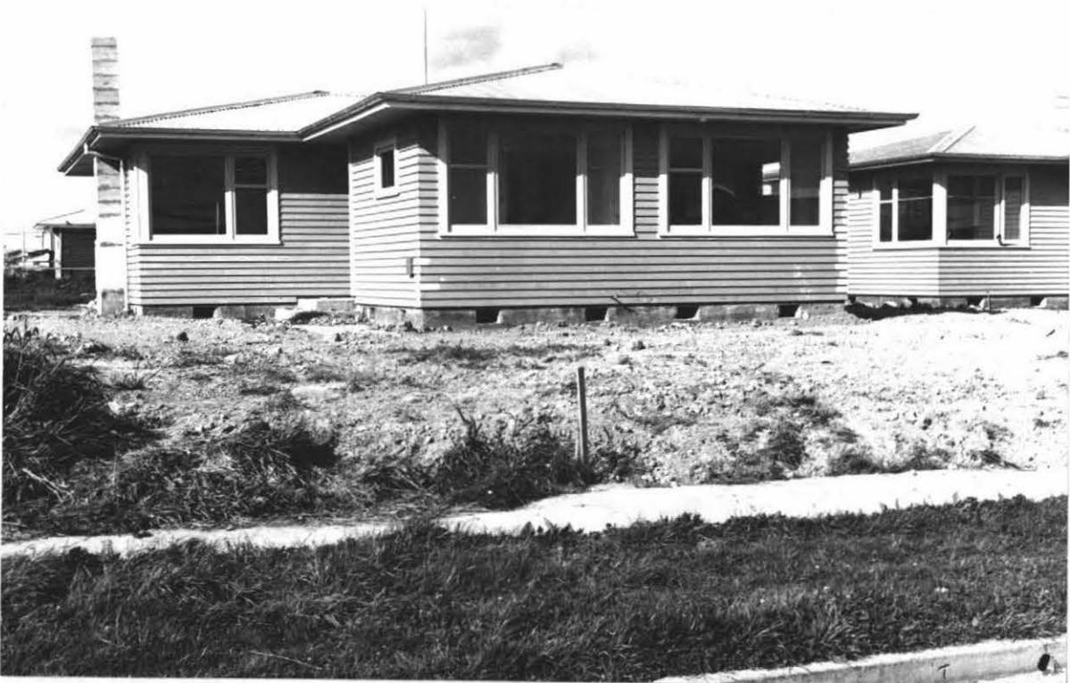
Figure 18. Group House Under Construction, Stephens Crescent.
