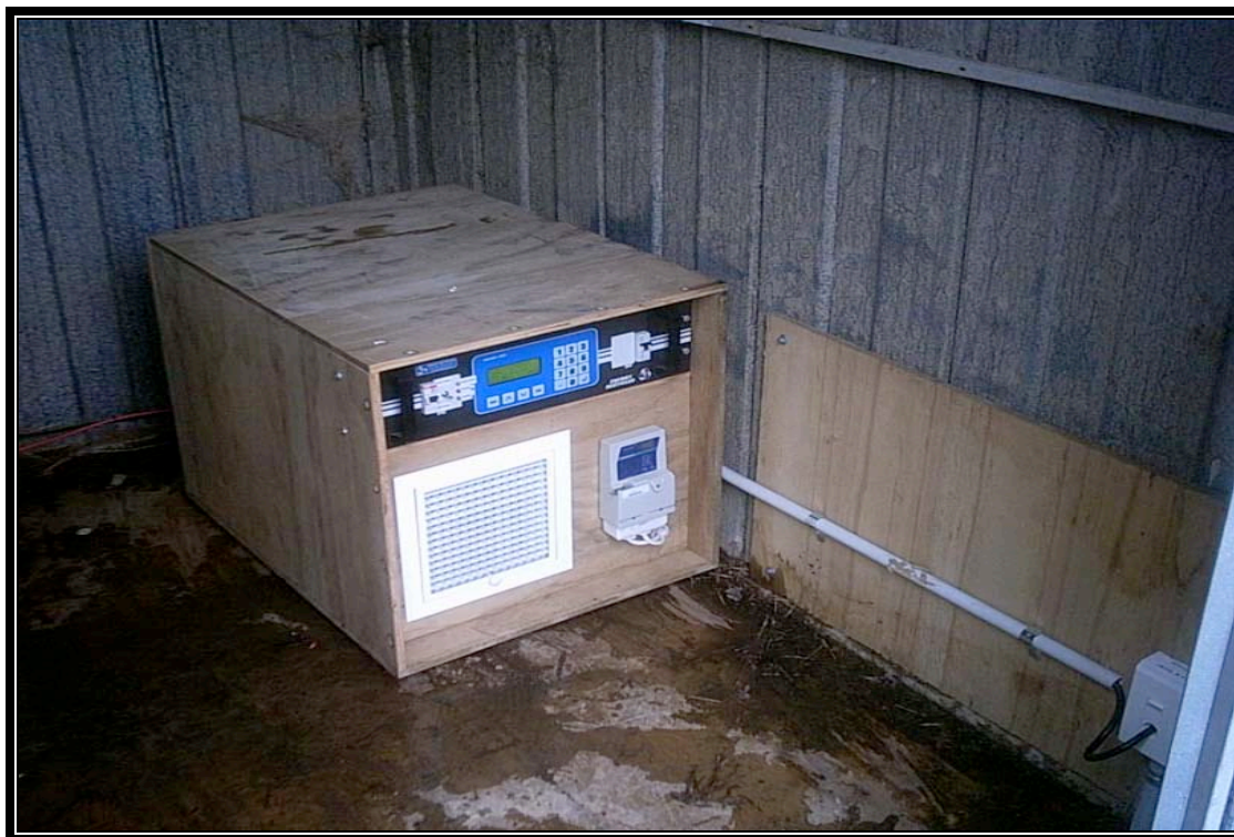
Figure 17 Energy Recyclers Inverter mounted in a protective cabinet
