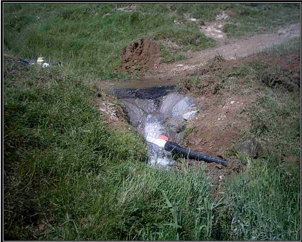
Figure 10 The intake assembly shortly after installation
