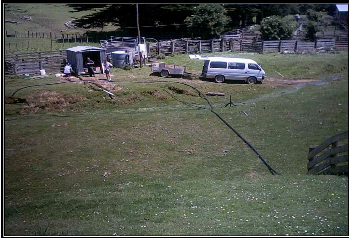
Figure 13 Turbine shed during construction
