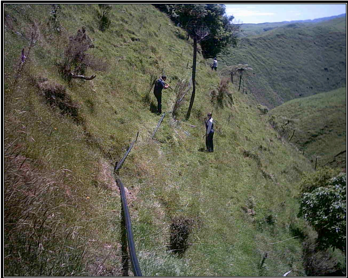
Figure 1 Installation of intake pipeline around a knoll 200m from intake site
