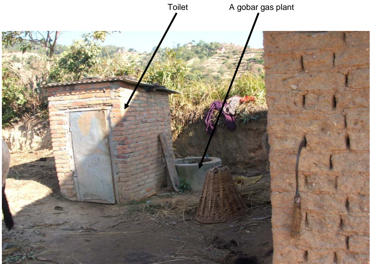
Figure 5.11: A gobar gas plant
