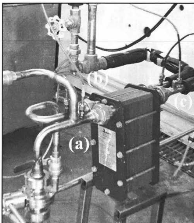
Figure 4.7 Plate heat exchanger and surrounding piping system (a) PHE (b) DSI that heated water used as heating medium for PHE (c) RTDs for heating medium inlet and process fluid outlet
