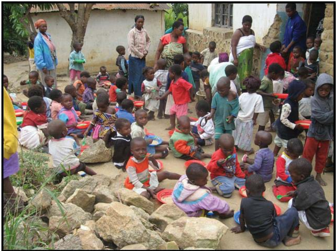
Figure 10: Orphans Being Fed Outside Due to the Leaky Roof
