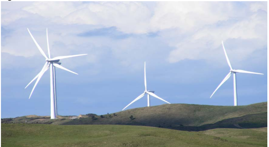
Figure A6.2 Tararua 3, 3MW Turbines
