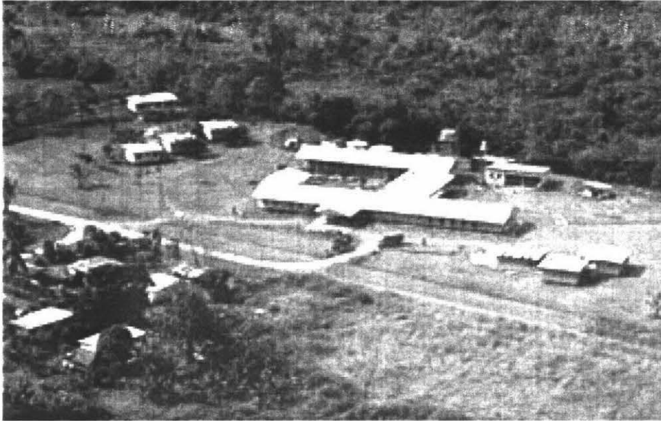
Figure. 4 Aerial view of Kokoda Memorial Hospital
